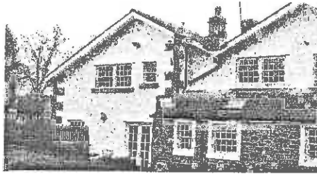
Figure 6: Rear extensions (built 2007)
