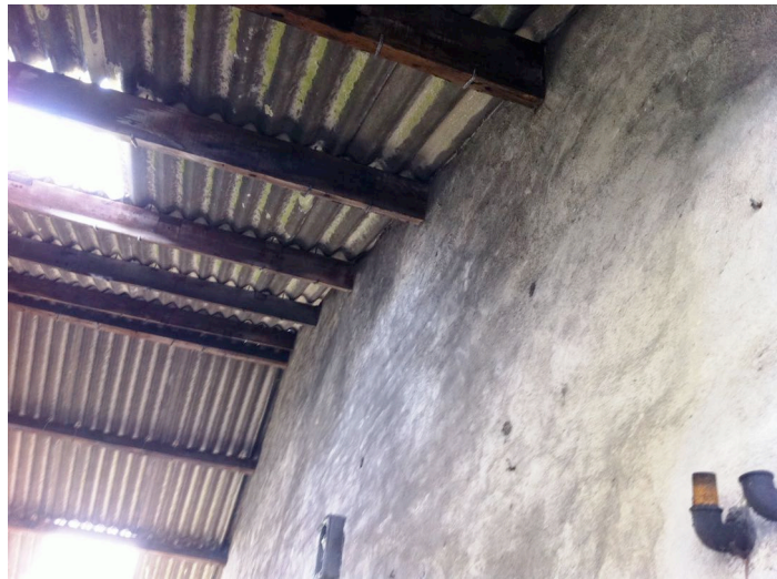
Photo 8. Detailed view of the roof underside of Internal view of the section of building proposed for removal, where it abuts the adjacent building section
