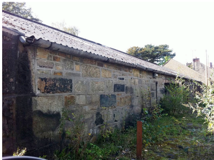
Photo 5. The front elevation of the section of building proposed for removal
