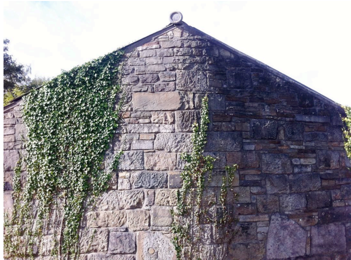
Photo 4. The gable end of the section of building proposed for removal
