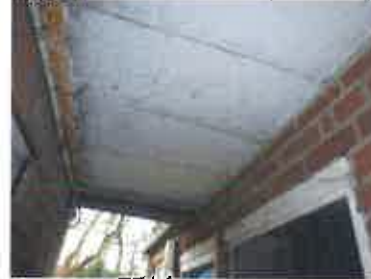
The section of roof connecting the house to garage
