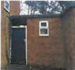
The walls are brick cavity construction.
