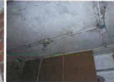
Internal view of roof in store
