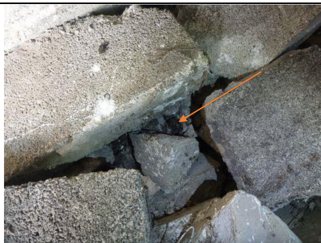
Photo 21: Building 1, old pellet under faecal splashing at central open section
