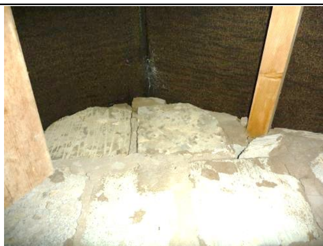
Photo 19: Building 1, assumed roosting position within western compartment
