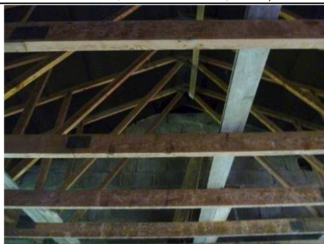
Photo 12: Building 1, internal area, eastern end of the building
