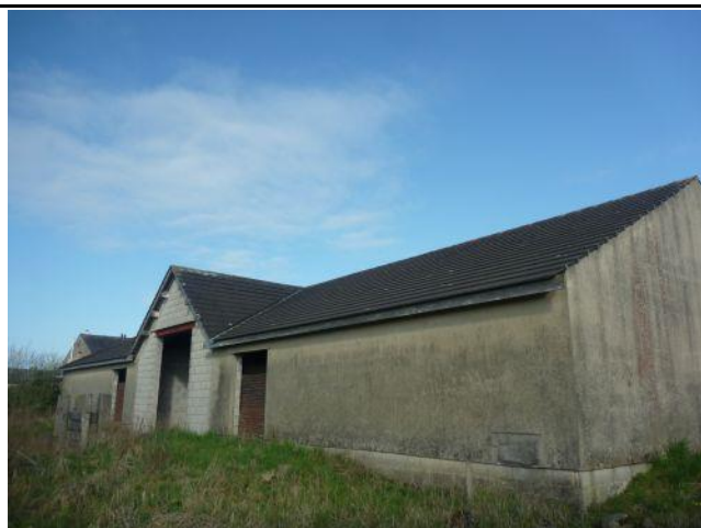
Photo 9: Building 1, southern elevation
