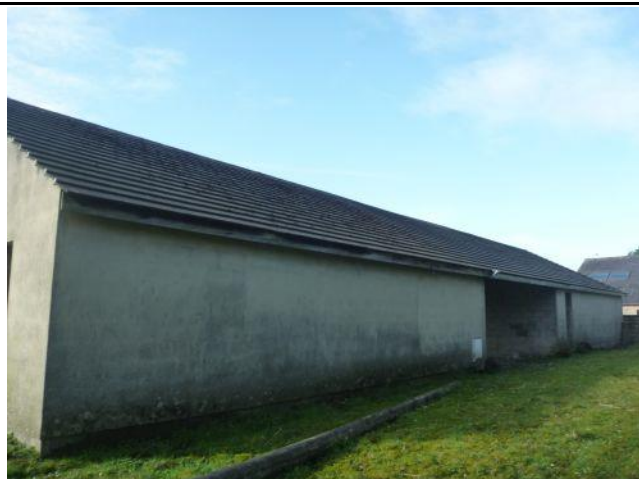
Photo 7: Building 1, northern elevation
