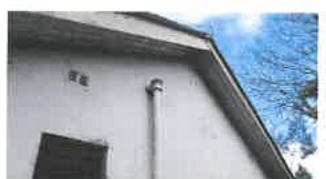
Figure 3: east gable end wall
