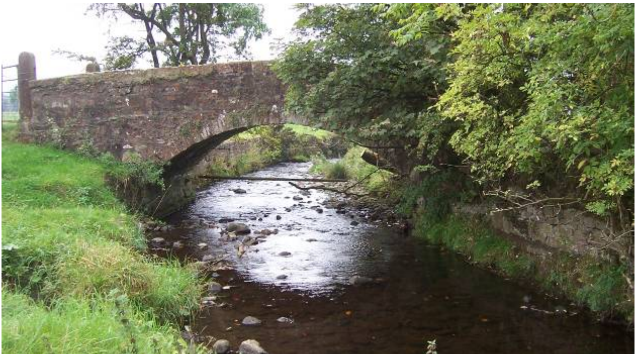
Northern elevation of the bridge
