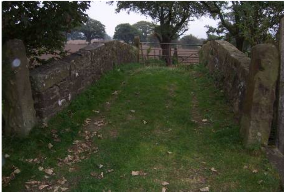
View of the bridge from Longridge Road (from west)
