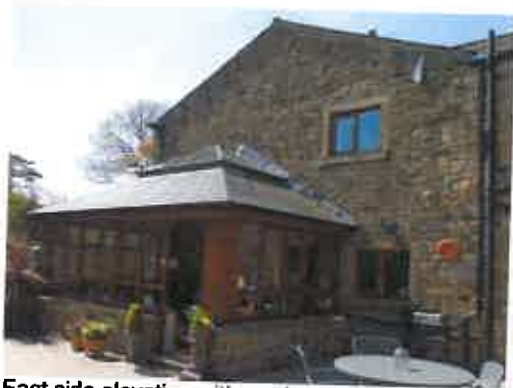
East side elevation with garden room extension
