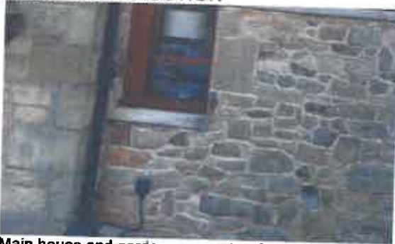
Main house and garden room extension wall.
