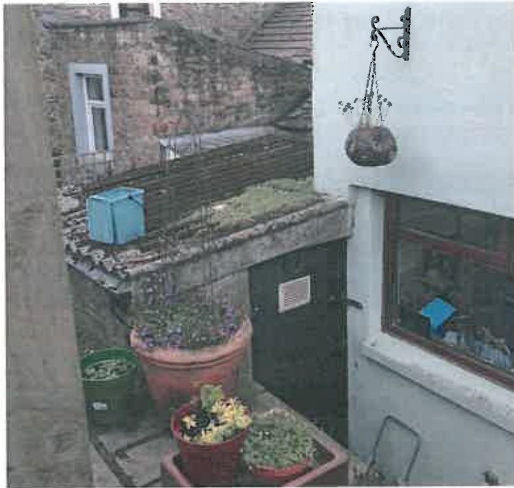
Single storey store attached to outrigger to rear
