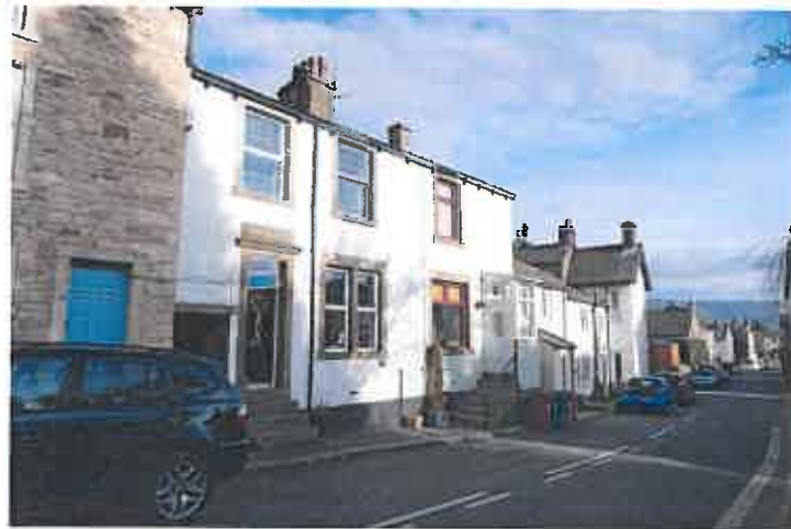
Street scene view to front elevation.
