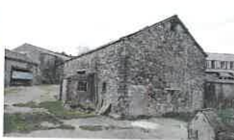
Figure 21: stone barn (east)
