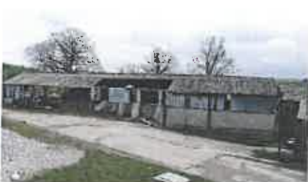
Figure 24: cubicle sheds (east)
