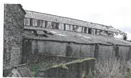
Figure 22: cubicle sheds (east)
