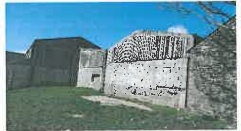
Figure 7: Cubicle sheds group 'A' at rear
