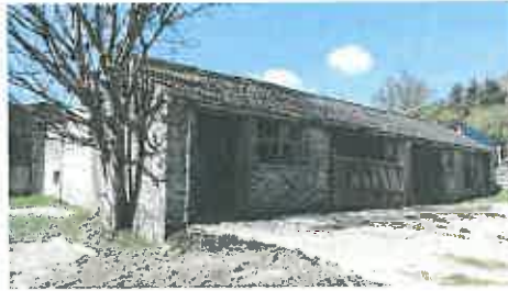
Figure 6: 4-bay shed – only one bay is closed
