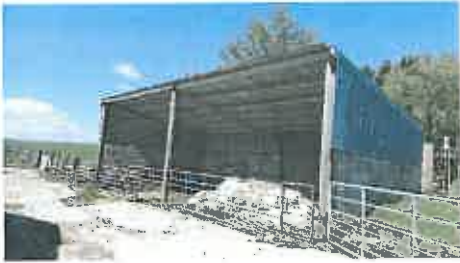
Figure 5: Open portal shed.
