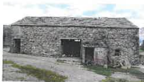
Figure 20: Stone barn (east)
