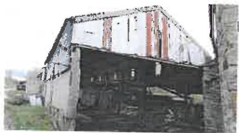
Figure 23: cubicle sheds (east)
