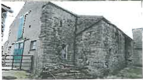
Figure 11: Stone shed / garage – group 'B'
