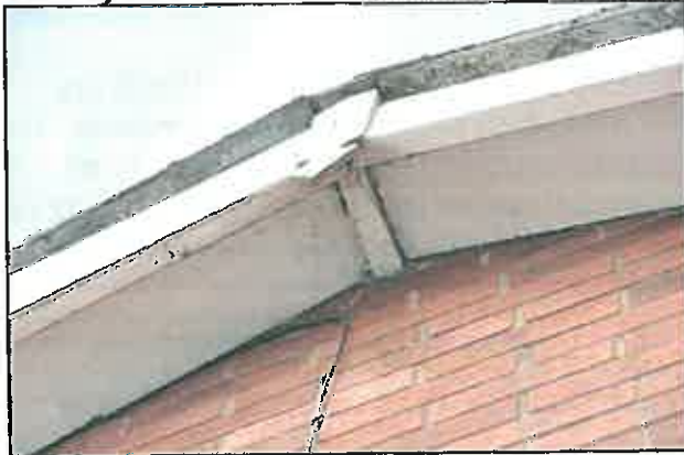
View of south gable with gaps between timber under boarding and brick wall (lhs) and internal view of roof showing ceilings have been removed (rhs)
