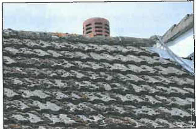
View of 61 Preston Road, west elevation (lhs) and close up view of tiles covered in moss (rhs)
