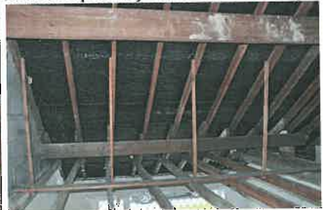
View of south gable with gaps between timber under boarding and brick wall (lhs) and internal view of roof showing ceilings have been removed (rhs)
