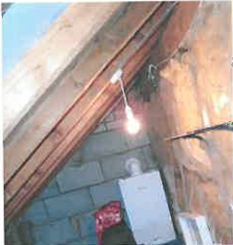
Roof space behind bedrooms.
