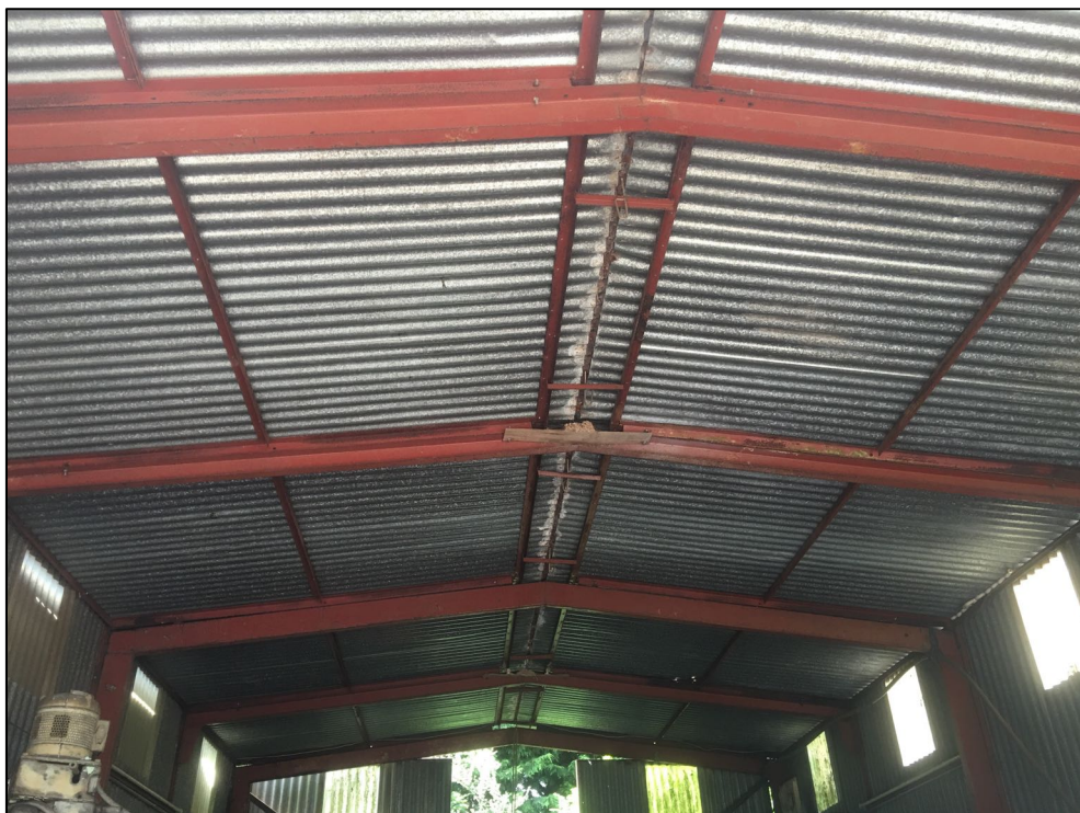
Figure 6 A typical internal view of one of the existing buildings
