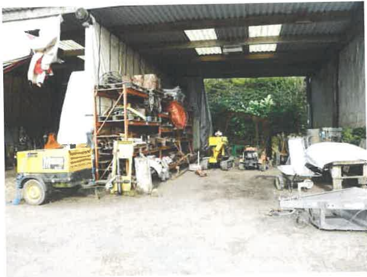
Photo 9 – Open workshop buildings within SE area, looking W.
