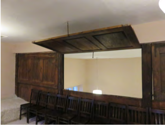
Gallery with opening timber hatches.
