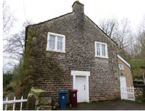
NE Elevation: Gable of Meeting room
