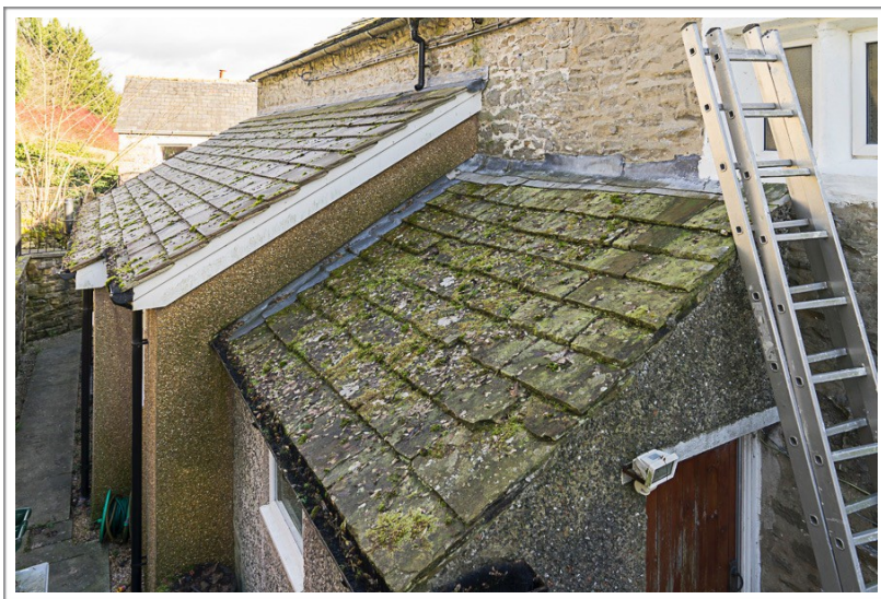
EXISTING EXTENSIONS TO THE REAR OF THE PROPERTY
