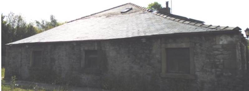
Lean to and hipped roof to the north west elevation.
