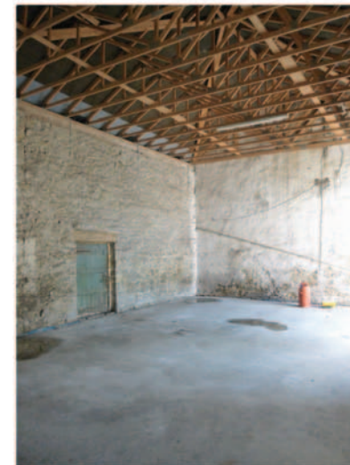
Current condition of the barn showing new roof construction
