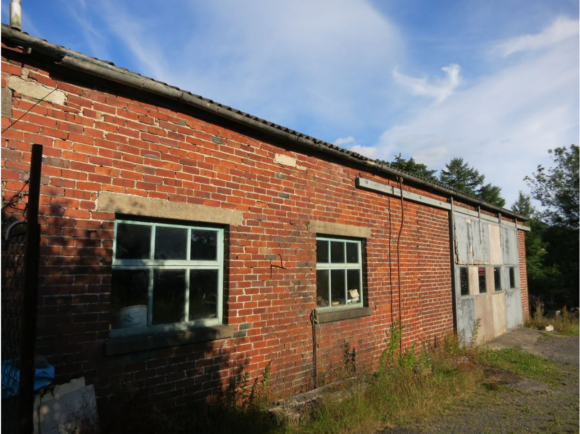
Brick built outbuilding with single skin roof
