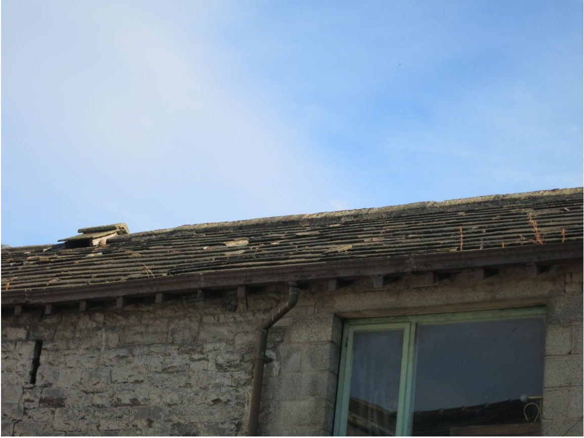
Roof of main barn
