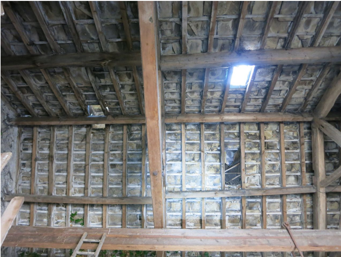
Roof of main barn
