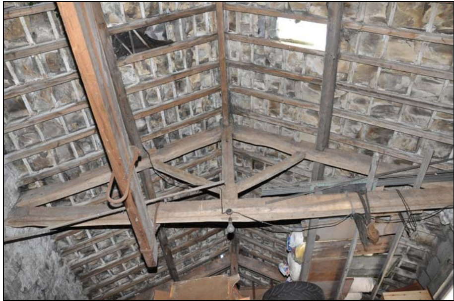
Former barn: underside of roof
