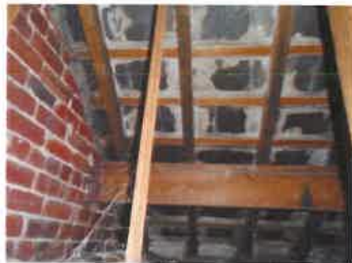
Second cottage roof void.
