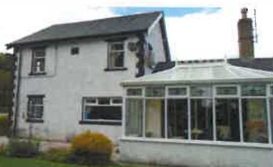
Main house and conservatory attached to the link.
