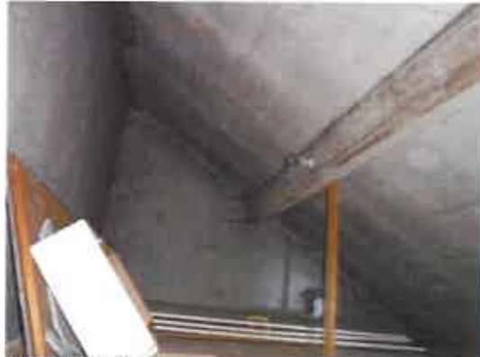
Main roof void.
