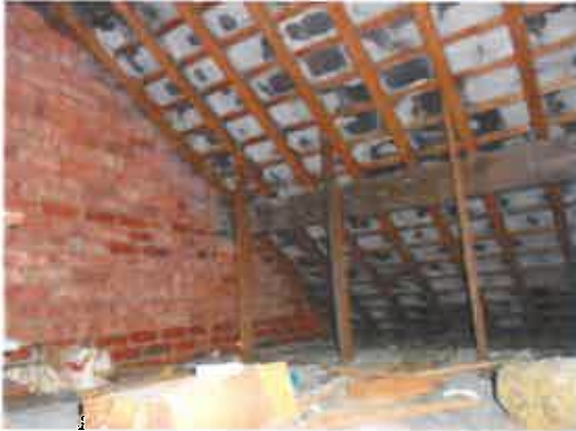
Main roof void
