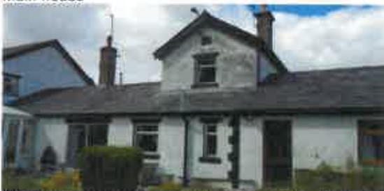
The link constructed around the original detached cottage.
