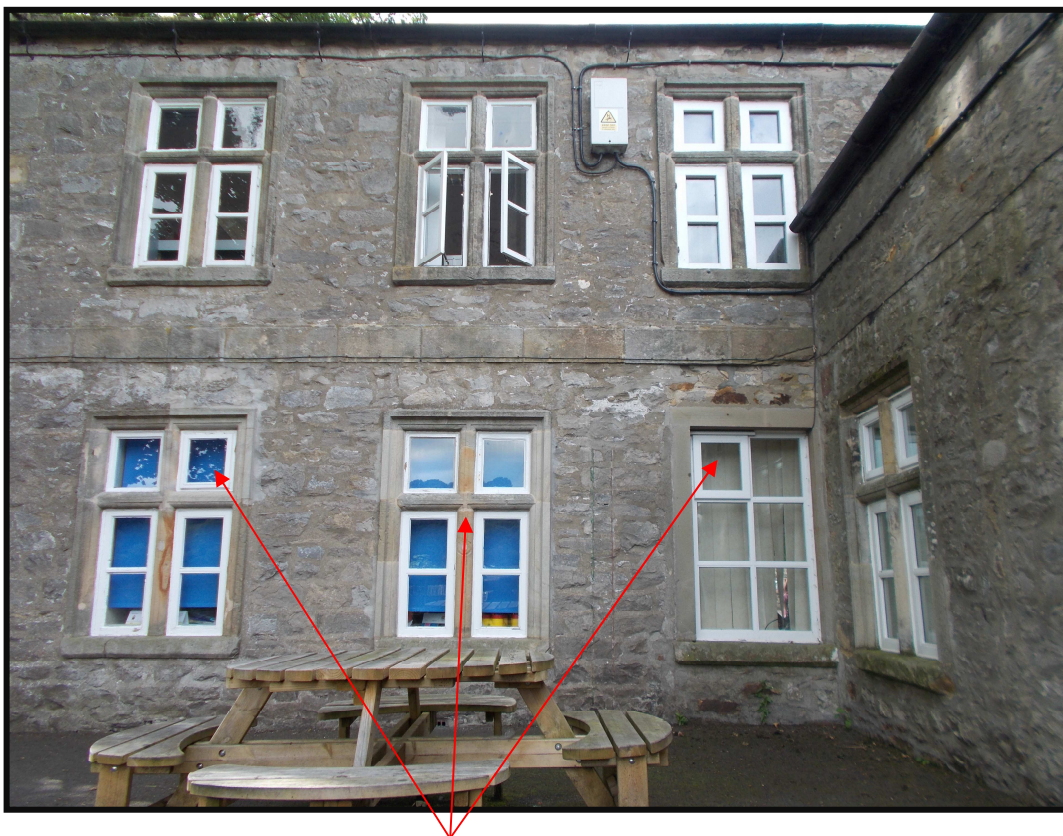
Windows to be refurbished and opening lights to be made operable
