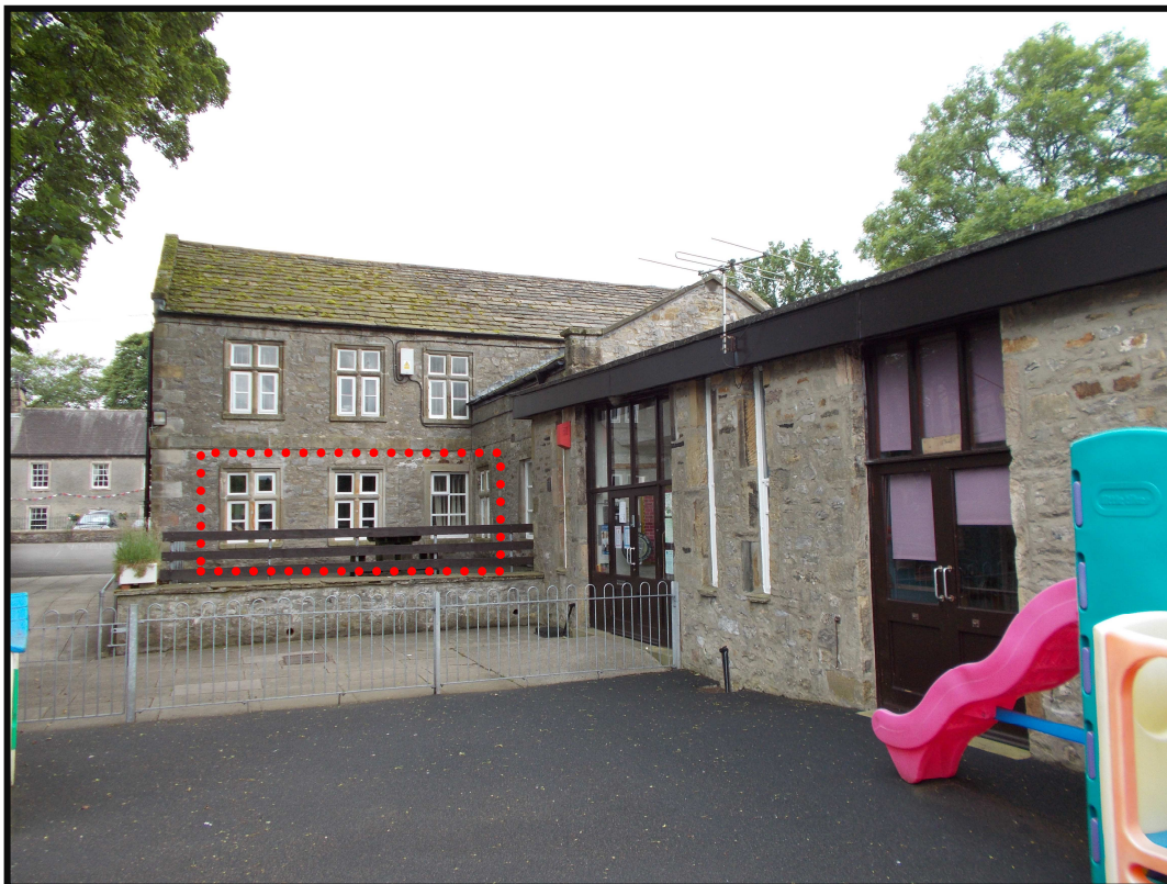
Figure 5 - Represents existing windows which are to be refurbished
