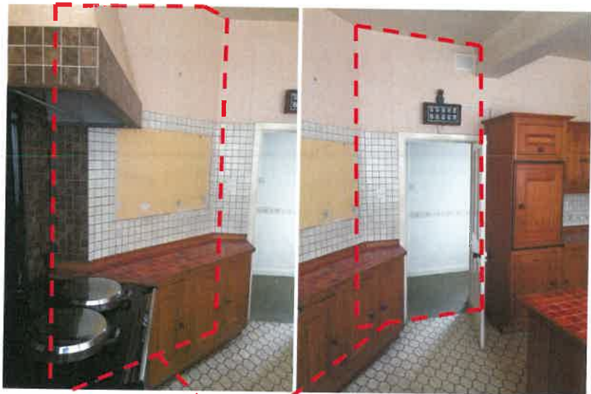
PL02 and PL03 (below) showing extent of sections of wall to be removed.
