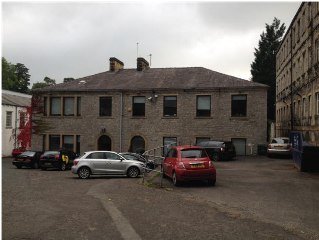
View of Primrose Mill Business Park to south of existing building
