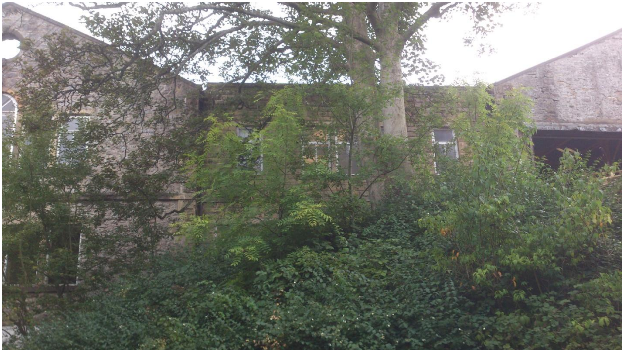
View of infill building between mill building and workshops.
