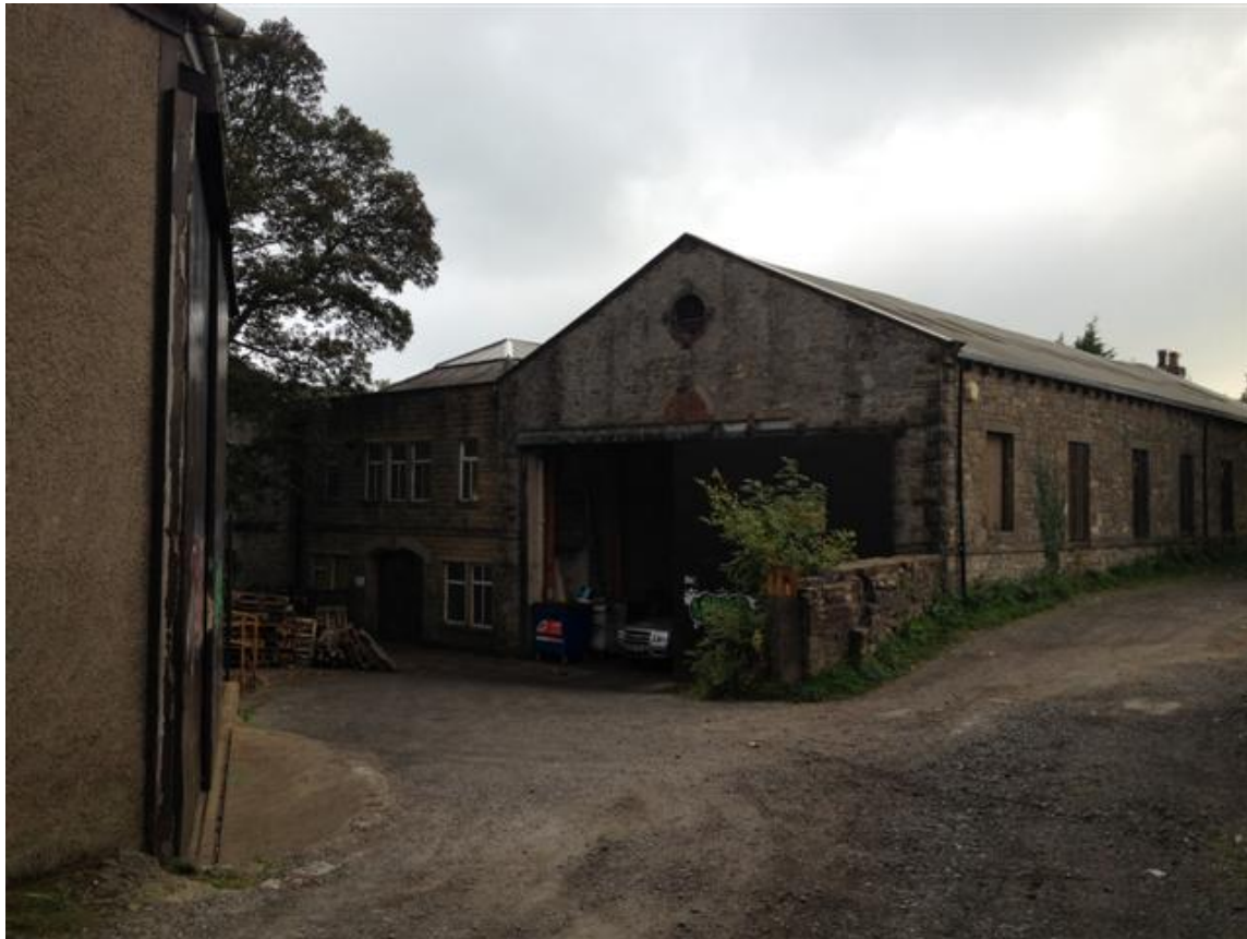
View of workshop building at upper level
