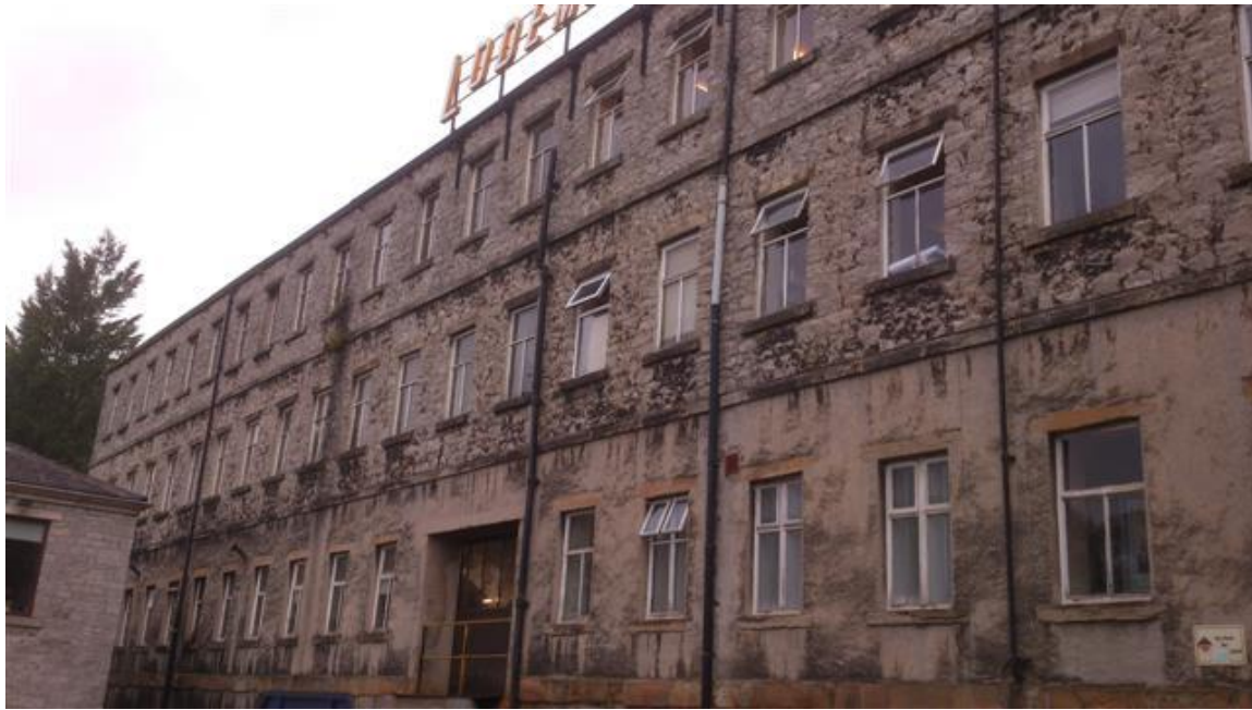
Rear elevation to existing mill building
