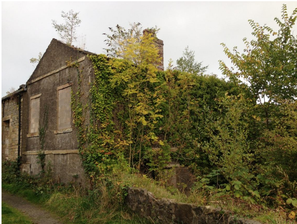
View of derelict cottage to rear of site.
