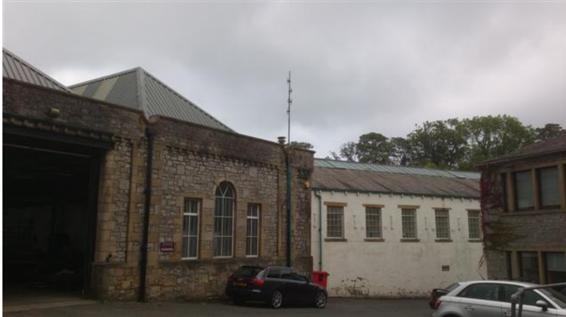
View of Primrose Mill Business Park to south of existing building
