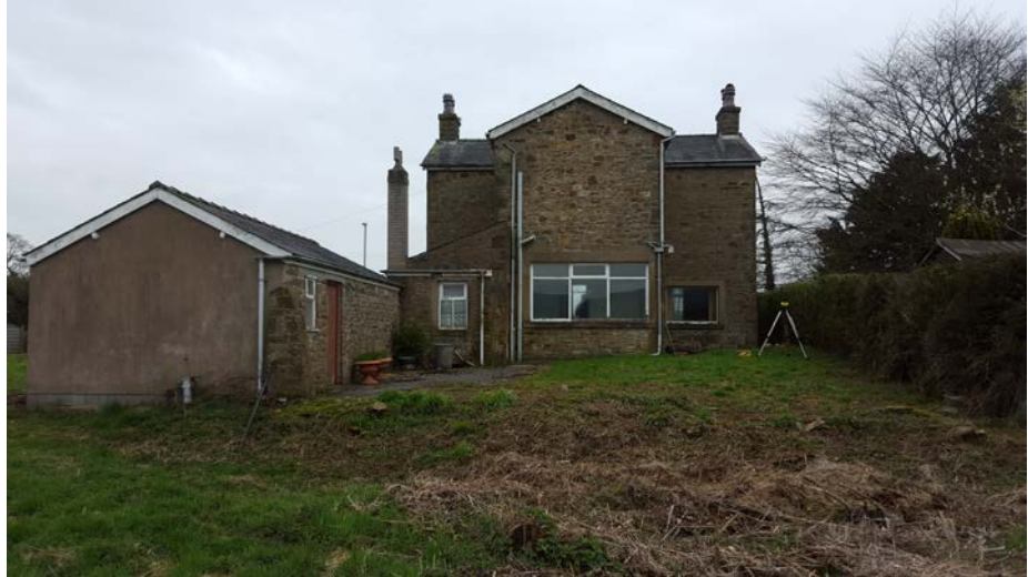
Figure 3 Rear 'outshoot' and garage to be demolished. Note only a few windows in rear
