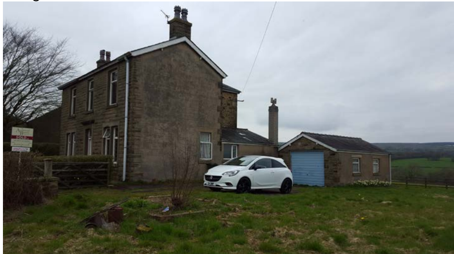
Figure 2 Photo from East of property with garage believed to be a later addition and everything else pretty much as originally built
