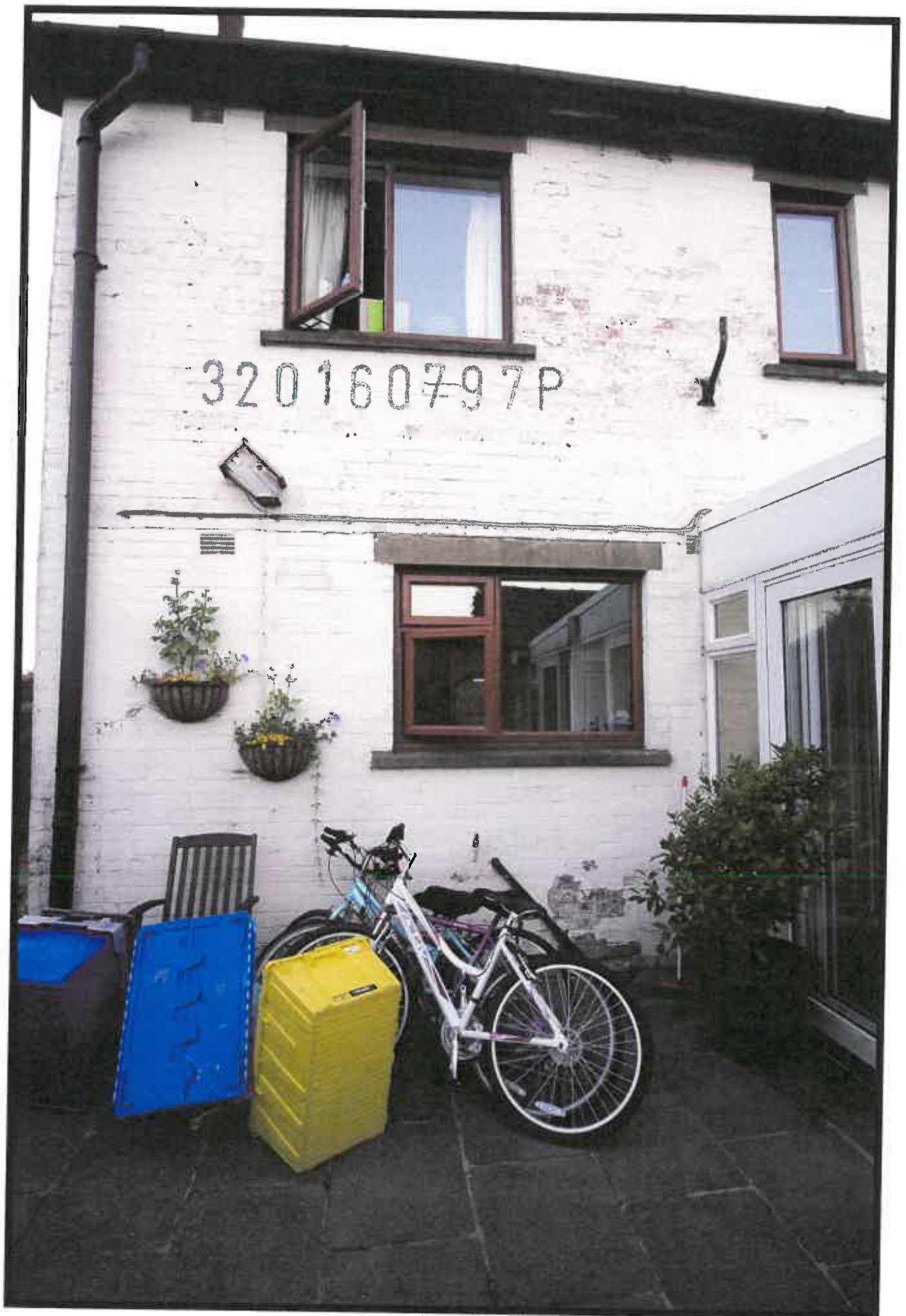
Site of the extension
