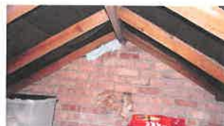
Figure 6: void 2 gable end wall
