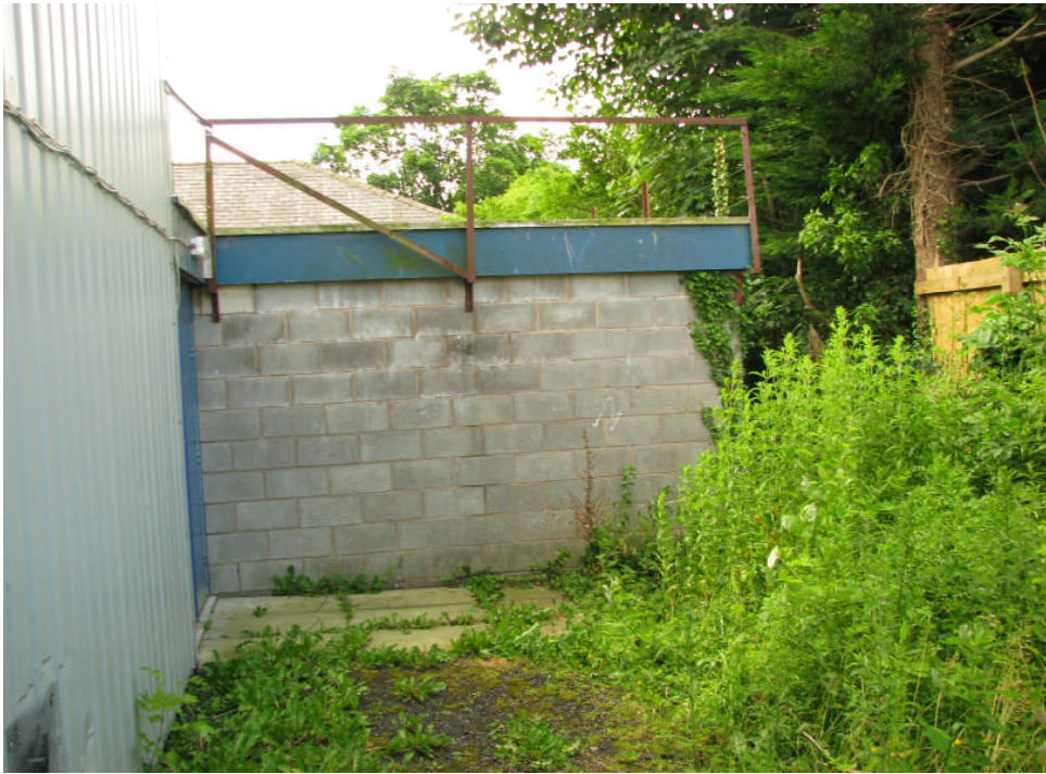
The existing changing room wall and rear service path
