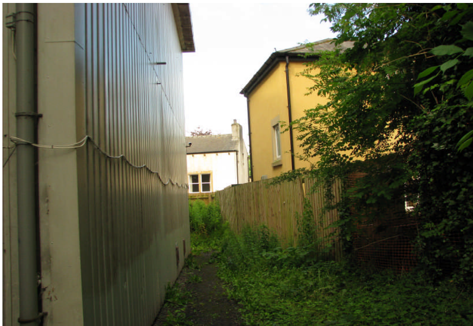
The rear fire escape route
