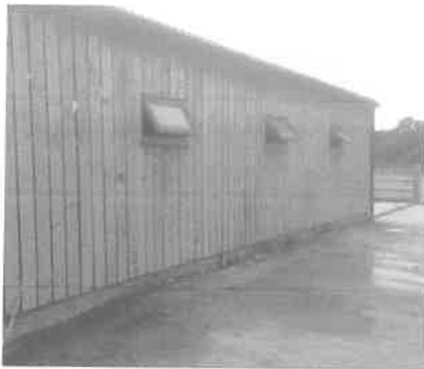
Existing stable building showing wood cladding. The proposed facilities block will use a similar vertical cladding system.
