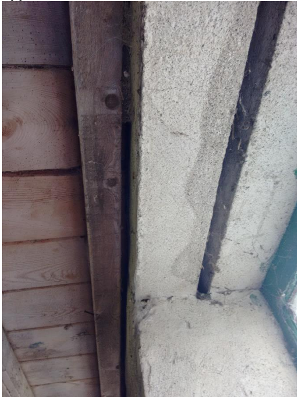
Photograph 9 shows the gap in the lintel and also between the upper timber floor and the lintel.
