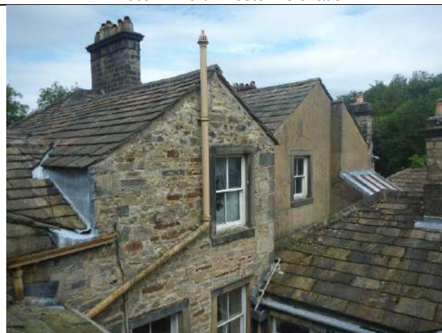
Photo 6: Complex rooftop, from south-eastern end looking north-west (view from bat activity survey position 2)
