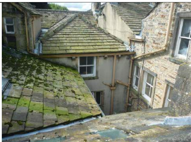
Photo 7: Complex rooftop, from northern-end looking south
