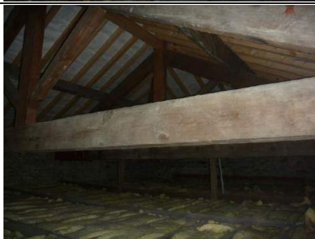
Photo 15: Roof Void D
