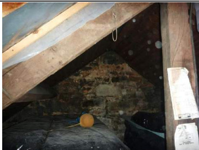
Photo 11: Roof Void B2 (middle/northern end) Separated from Roof Void B1 via plastic sheeting. Dimensions: 2.5 metres tall, 7.5 metres wide by 5 metres long. Construction type and materials: As per B1. Covered water tanks are present. The roofing is lined by timber planks. Signs of roosting bats Occasional scattered droppings, indicative of bats in flight present. No bats or signs of roosting bats present.
