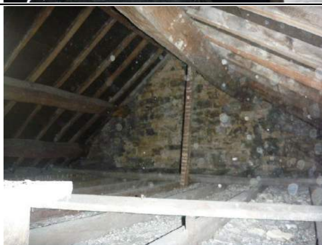
Photo 12: Roof Void B3 (middle/southern end) Dimensions: 2.5 metres tall, 7.5 metres wide by 5 metres long. Construction type and materials: Constructed from traditional timber purlins and rafters. Roofing slates lined with bitumastic roofing felt. Floor is uninsulated. Signs of roosting bats 100's of droppings (of a size and shape indicative of pipistrelle species) distributed under the ridge line. No bats detected. Roost 4, refer to Photo 28, Table 8.3.
