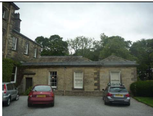
Photo 2: Single-storey extension at north-eastern end
