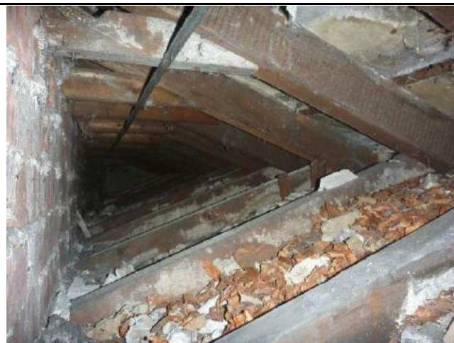
Photo 19: Roof void H
