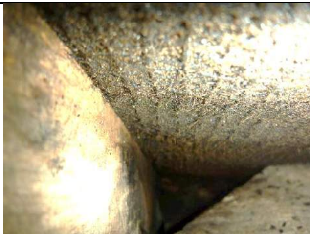
Photo 25: Roost 1 roosting location at eaves.
