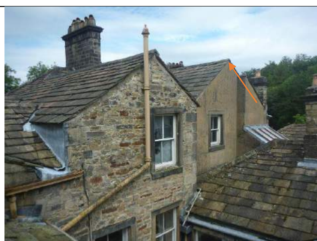
Photo 39: Roost 7 emergence and re-entry location
