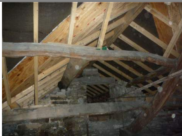
Photo 14: Roof void C
