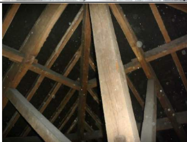
Photo 13: Roof Void B4 (southern end) Dimensions: 2.5 metres tall, 7.5 metres wide by 5 metres long. Construction type and materials: Hipped end. Constructed from traditional timber purlins and rafters. Roofing slates lined with bitumastic roofing felt. Fibreglass insulation present at floor. Signs of roosting bats 10's of droppings detected scattered within void, indicative of bats in flight. Cluster of 50+ droppings present under ridge-line. Roost 5, refer to Photo 29, Table 8.3.
