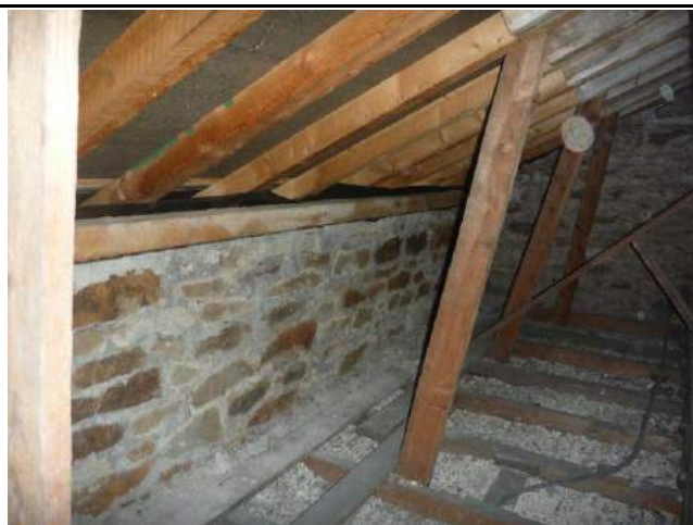
Photo 16: Roof void E
