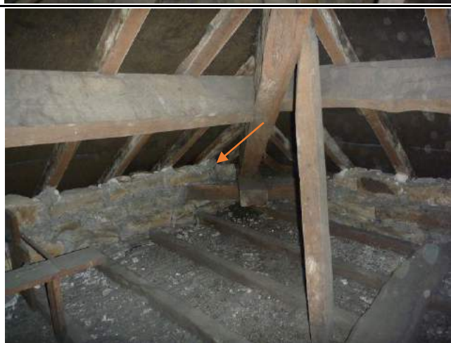
Photo 10: Roof Void B1 (northern end)
