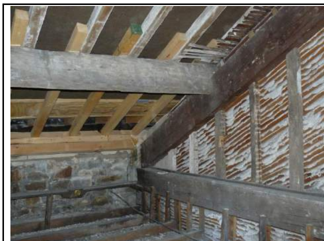
Photo 17: Roof void F
