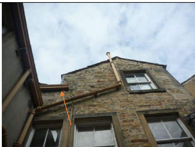
Photo 40: Roost 11 re-entry location
