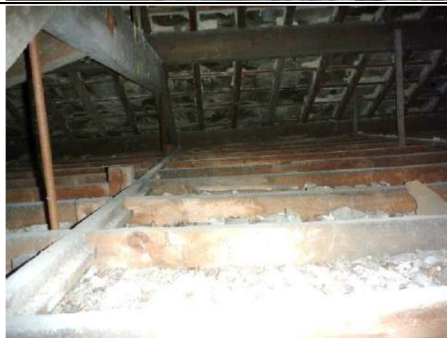
Photo 18: Roof void G
