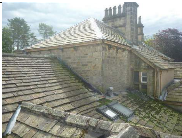
Photo 8: Complex rooftop, from north-western end looking south-east (view from bat activity survey position 1)
