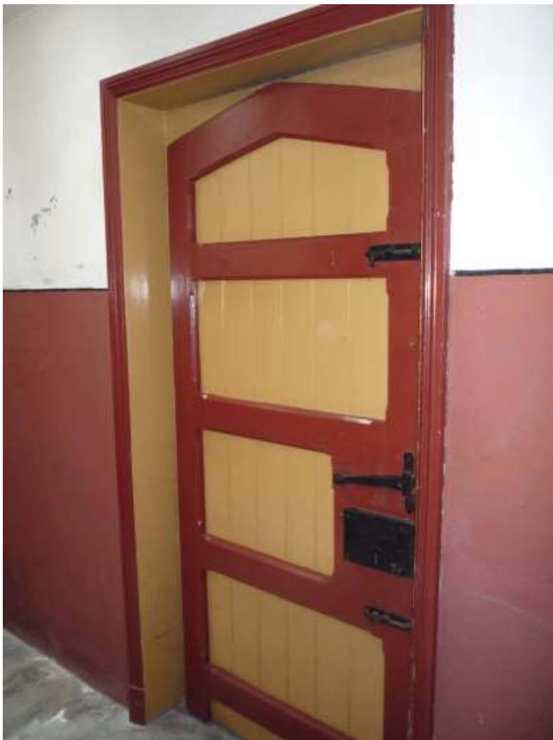
11. Re-used door leading to inner yard from 1892 cross passage.
