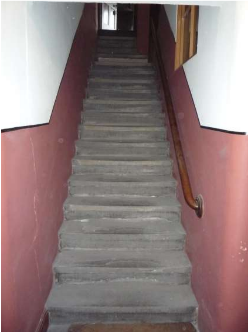
12. Staircase from ground to first floor inserted in former laundry range in 1892 view from G9g.
