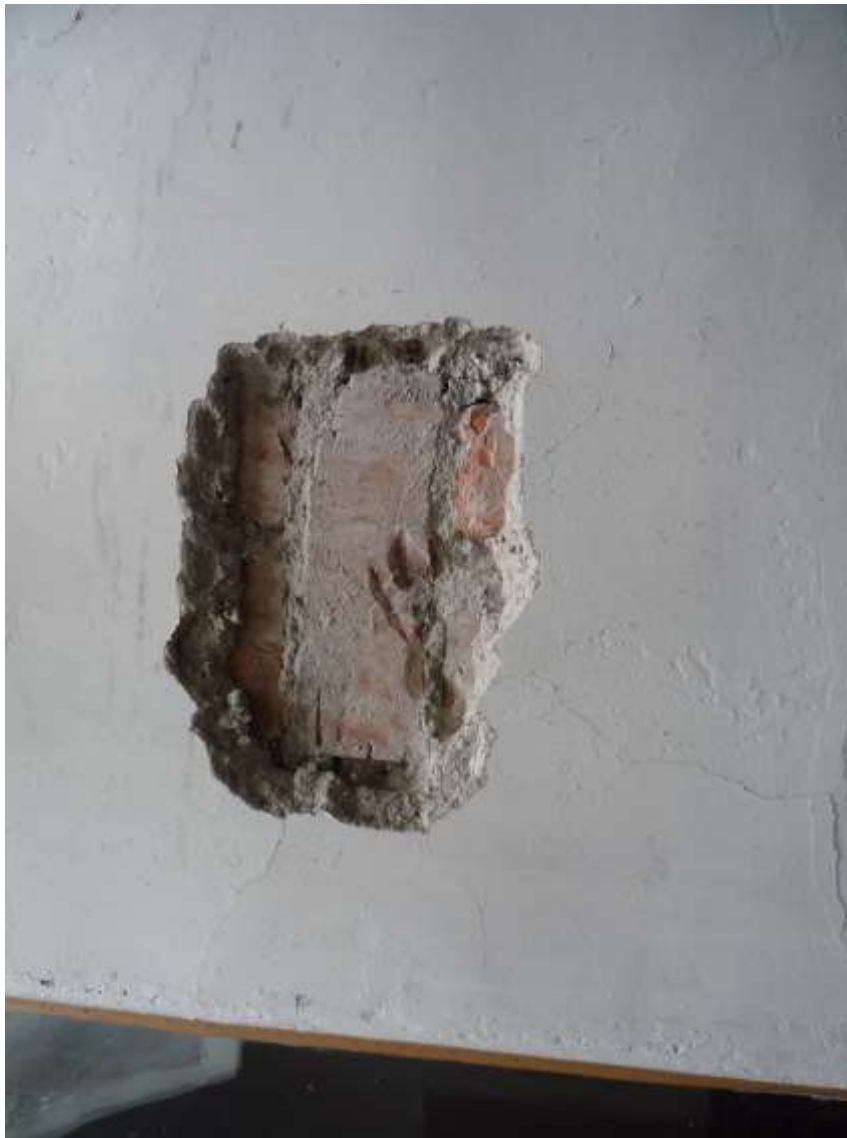
8. Investigations under plaster of the former laundry range ground floor south wall, revealing 1892 brickwork (G9a).
