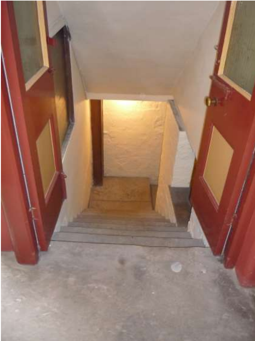
6. Stone flight to cellars in the former laundry range. To be retained in situ and floored over. Viewed from G9b.
