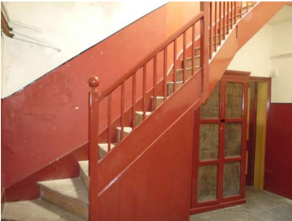
7. Simple Victorian back stairs (off G13). One of five service stairs in the house. To be removed.
