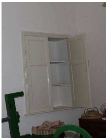
Plate 61: Pair of two-panel cupboard doors fitted to a built-in wall cupboard. Lower panels larger than upper panels, which are nearly square, all with moulded margins. Modern upright handle fitted to west door. Late 19th century
