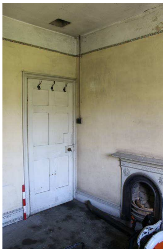
Plate 45: Room F19a , facing south-east, 0.5m scale
