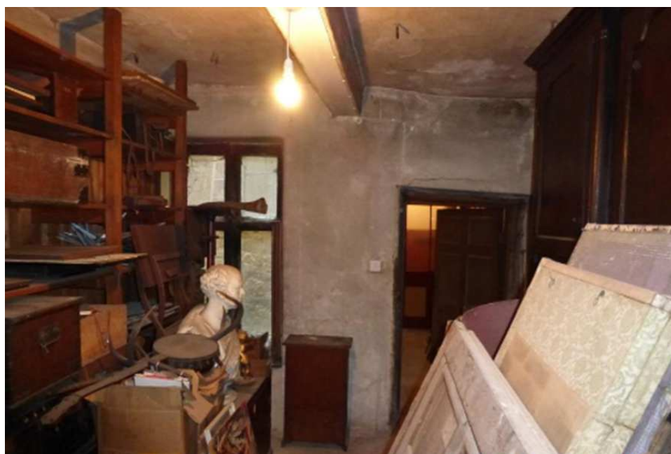
Plate 15: Room G27a facing north
