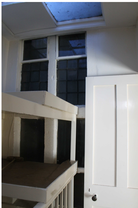
Plate 32: Mullion and transom window in Room F14i
