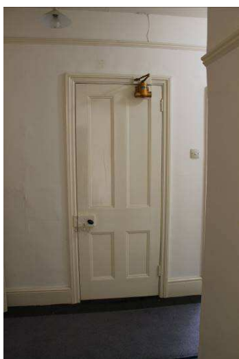
Plate 92: Four-panel timber door, with moulded margins. Upper panels larger than lower panels. Hinged to the east, with ovoid brass door knobs, locking plate on the south face over a draw bolt. Late 19th century.
