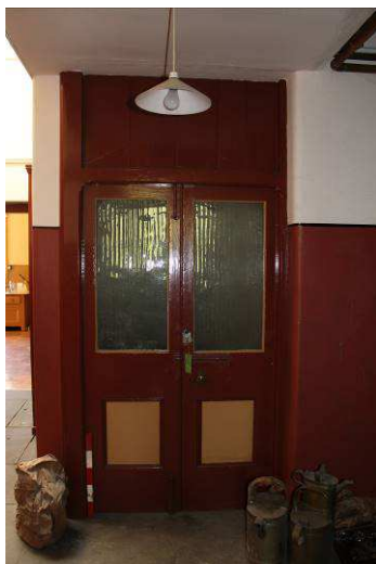
Plate 62: Pair of double timber doors, each with large glazed upper panel fitted with fluted glass and smaller lower panel, both with moulded margins. Hinged to the north and south, with brass knob fitted to south door and vertical draw bolts to north door. Late 19th century
