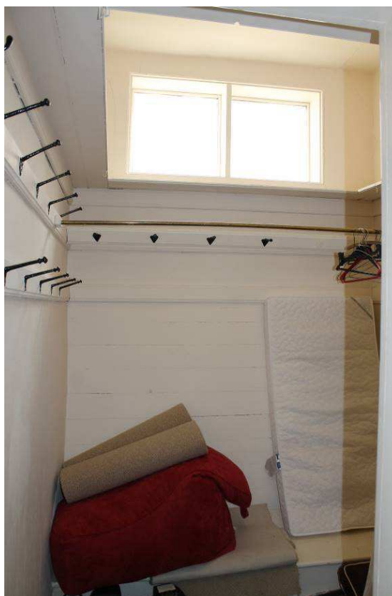
Plate 34: Cupboard Room F20 , facing east
