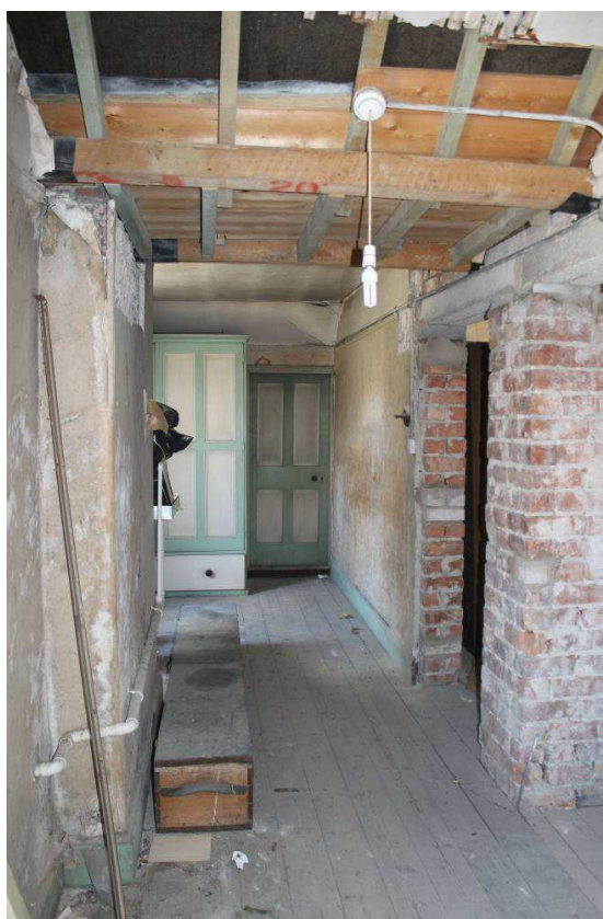
Plate 35: Corridor Room S3 , facing south
