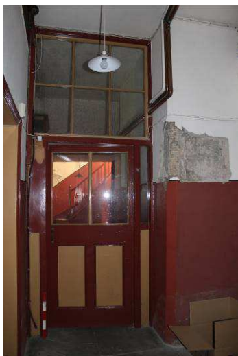
Plate 58: Four panel timber door, lower panels with moulded margins, upper panels slightly wider and glazed with slender narrow mullion between. Hinged to east with wrought iron upright handle on north side. Narrow side-light to east and six panel over-lighter arranged in two rows of three. Late 19th century
