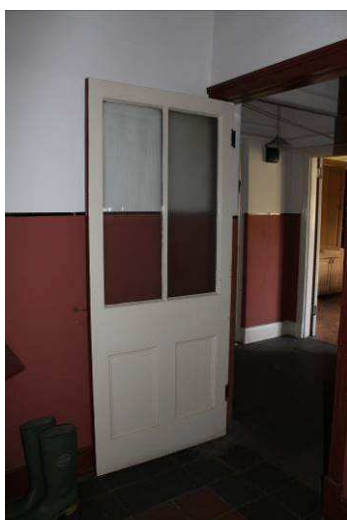
Plate 66: Four-panel timber door, with moulded margins. Hinged to the west, with larger fluted glazed upper lights separated by a narrow mullion. Late 19th century
