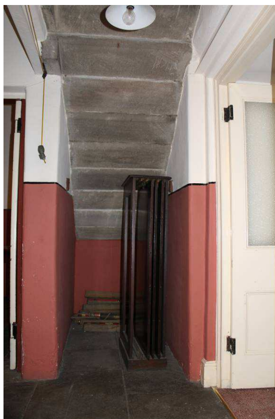
Plate 12: Room G9d , facing south
