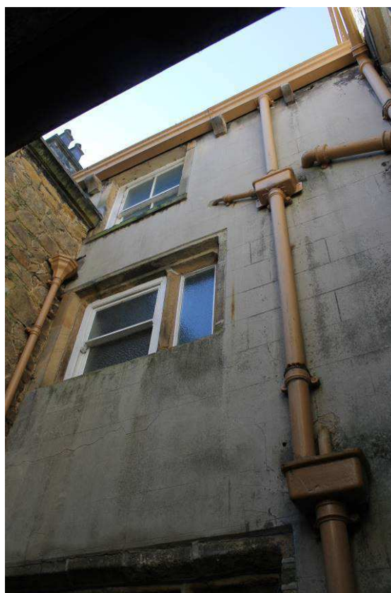
Plate 18: South wall of central yard
