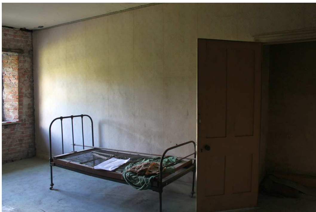
Plate 50: Room F21b, facing south-east
