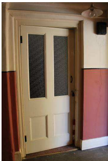
Plate 64: Four-panel timber door with two larger glazed panels above two smaller panels, all with moulded margins. Textured glass, hinged to the south with upright iron handle on east and west faces. Late 19th century
