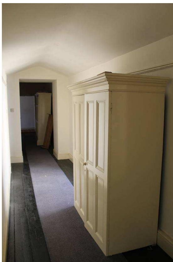
Plate 29: Corridor Room F14f , facing south
