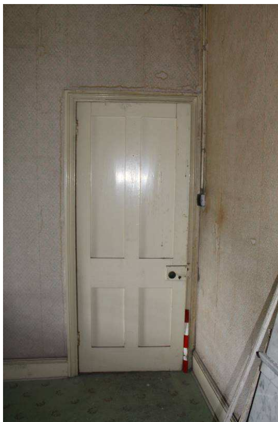
Plate 51: Room F21b, facing south, 0.5m scale
