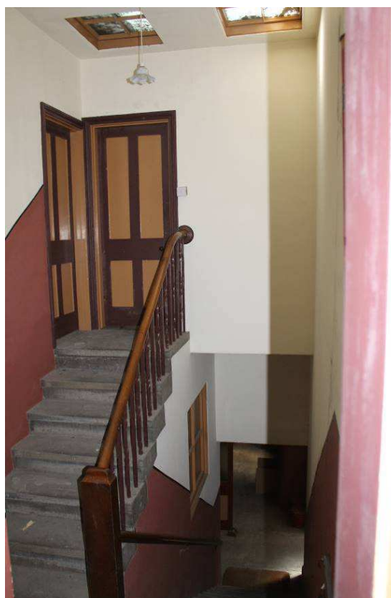
Plate 30: Stairwell Room F14g , facing south
