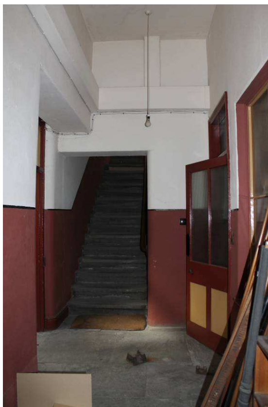
Plate 14: Room G9g , facing north
