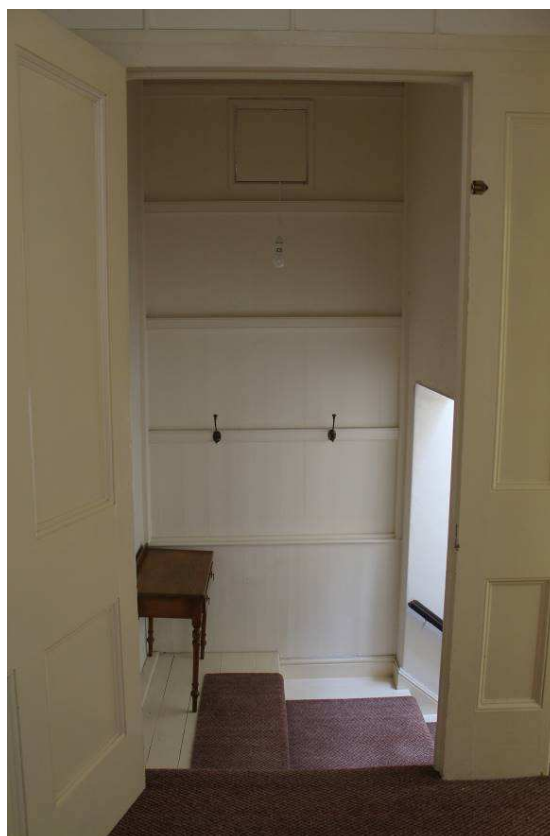
Plate 26: First floor landing at top of staircase Room F14c , facing north
