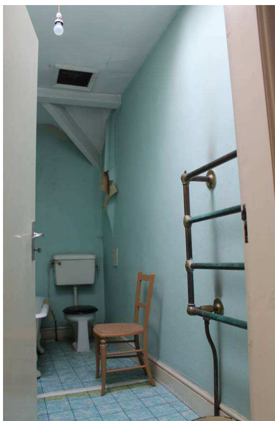
Plate 31: Room F14h , facing north
