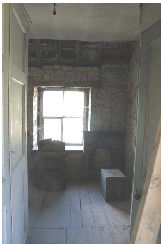
Plate 36: Room S9 , facing north
