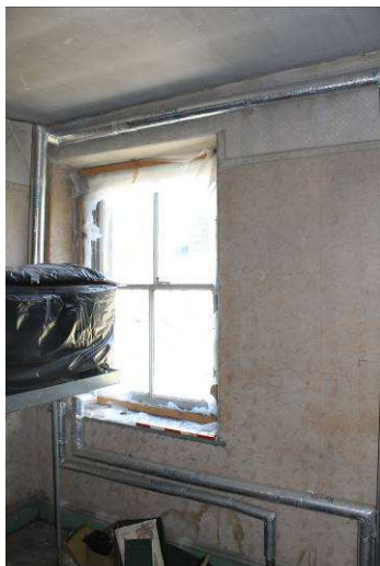
Plate 111: Two-over-two light timber sash window. Plain square section external stone surrounds, not closely inspected but appear similar to those on the floor below. Sash fastener on interior meeting rail. Late 19th century.
