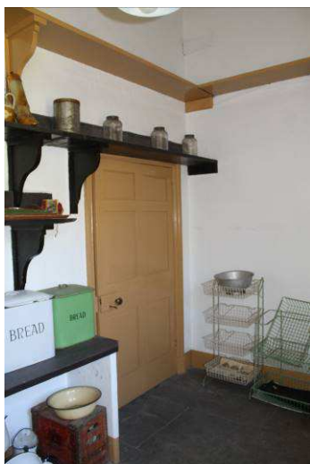
Plate 63: Short six-panel timber door, with smallest panels at the top. Hinged to the north with locking plate on east face and brass knob. Early 19th century
