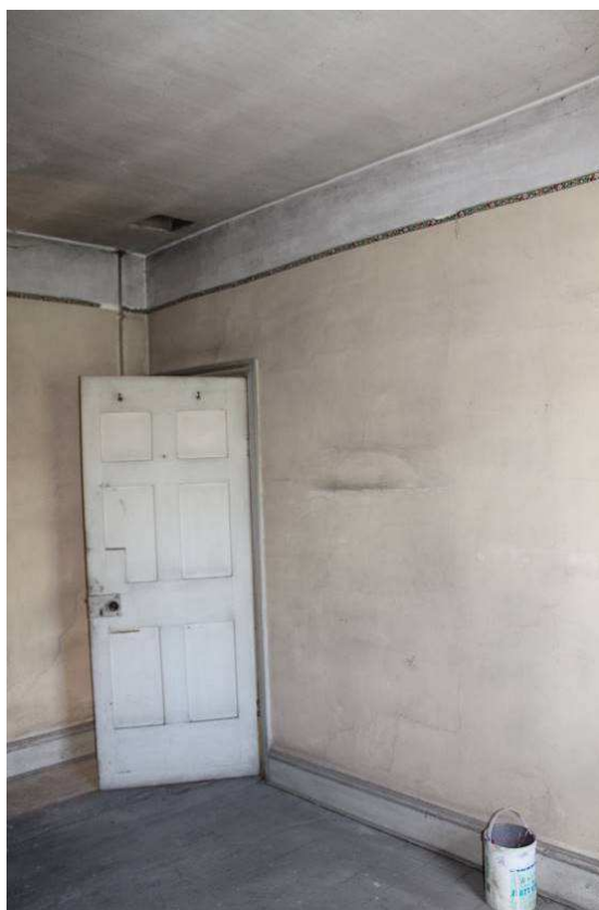
Plate 47: Room F19b, facing south-east
