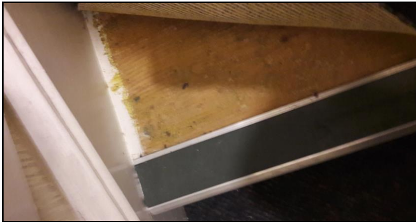
Figure 2. Modern softwood stair tread beneath carpet
