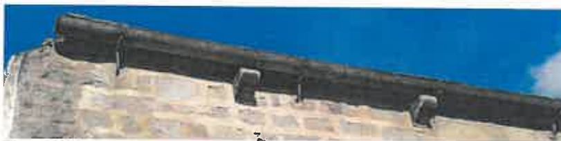
The gutters are mounted on brackets.
