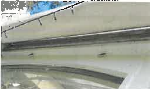
The gutters are mounted on brackets.
