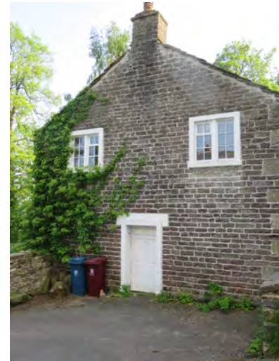
Current parking area alongside North East gable elevation.
