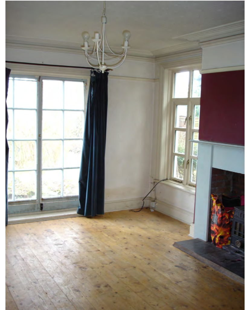
Cottage Dining Room showing the side gable window opening, where proposed link through to new Garden Room will be made.
