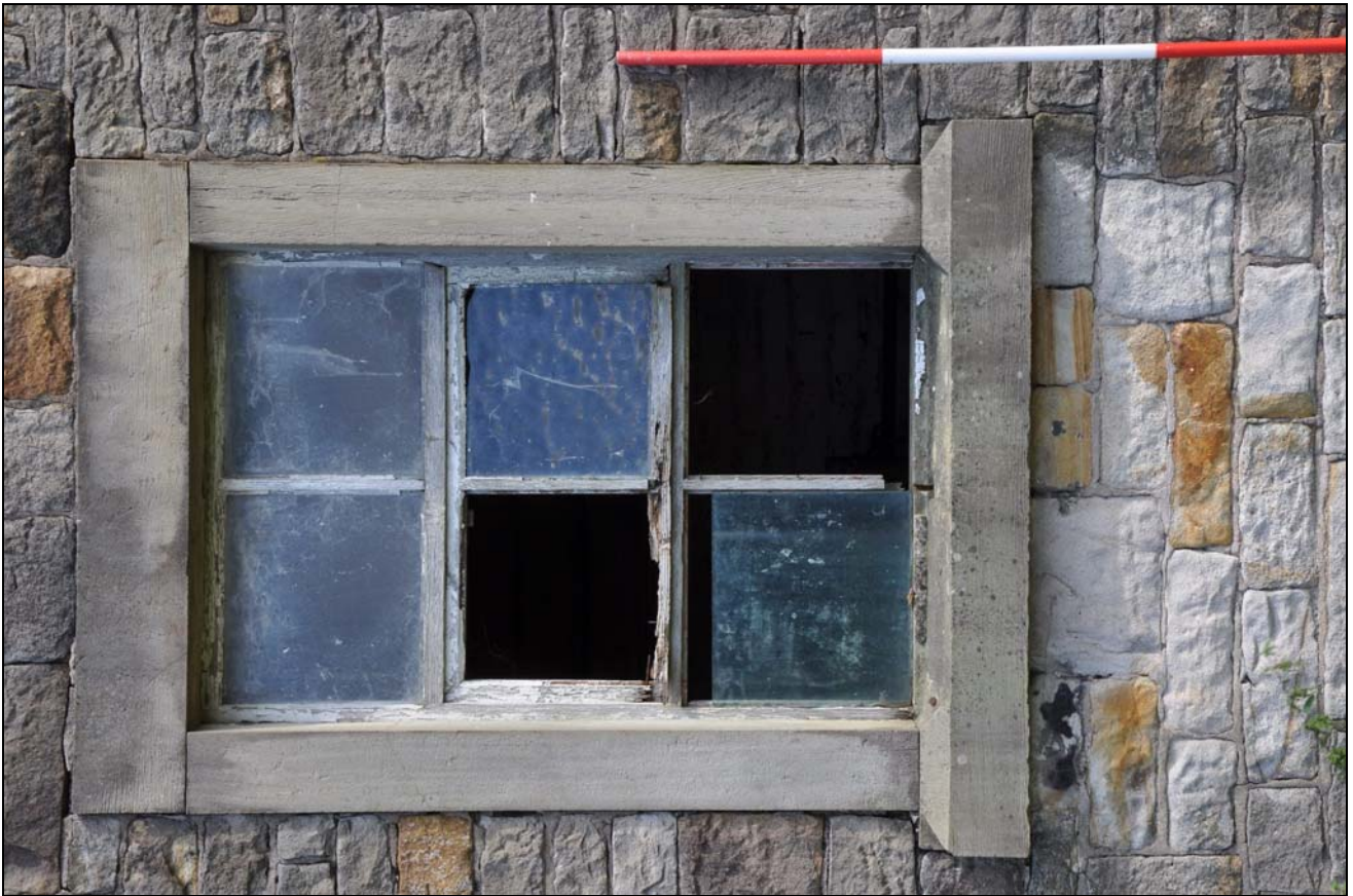
Photo 17: Detail of window, south-west side of barn
