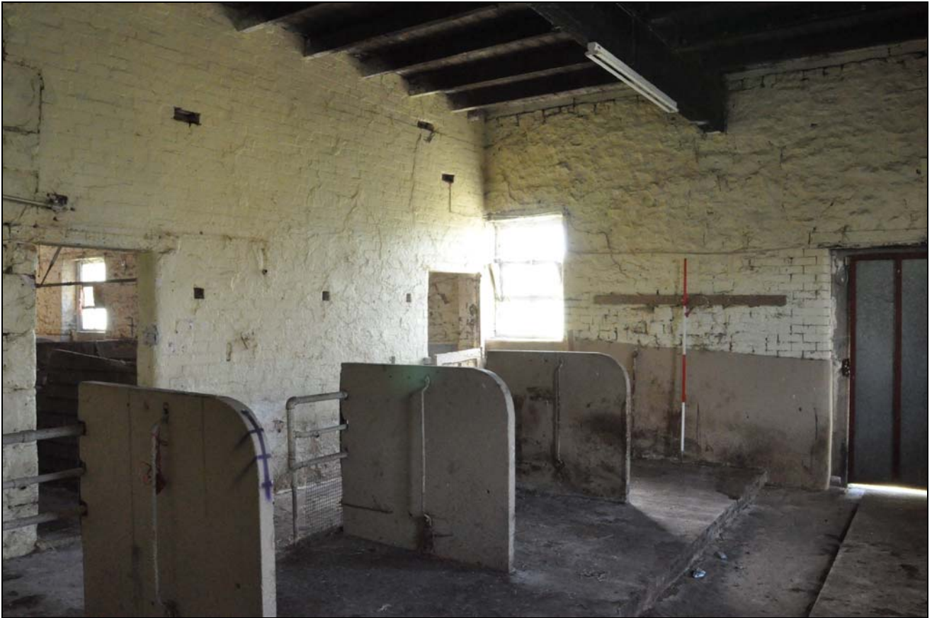
Photo 24: Small shippon in north-west end of barn, from the north
