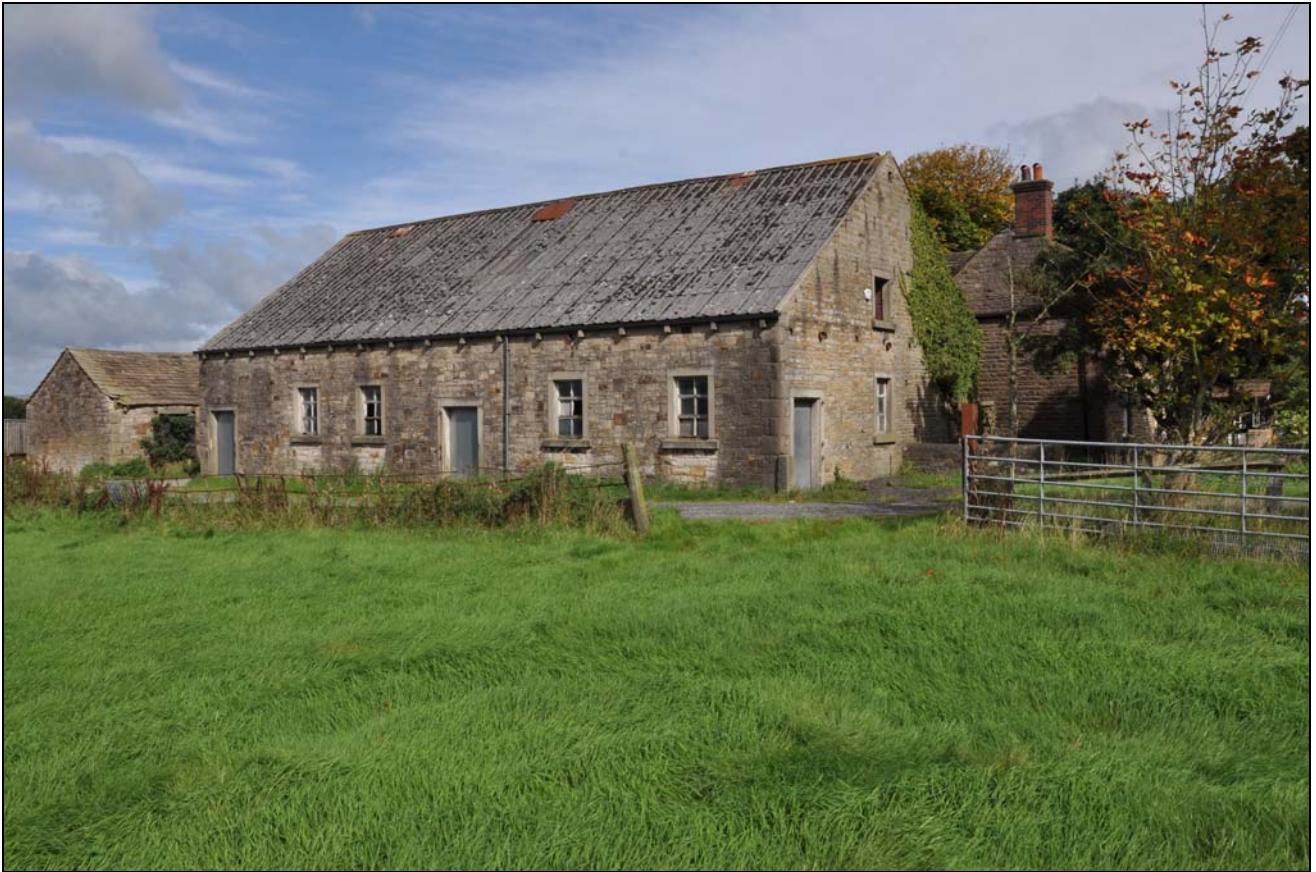
Photo 1: General view of the buildings, from the south-west
