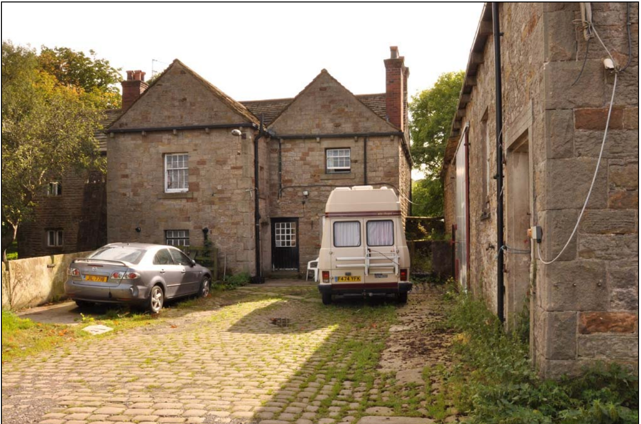
Photo 6: Rear of farmhouse and north-east side of barn
