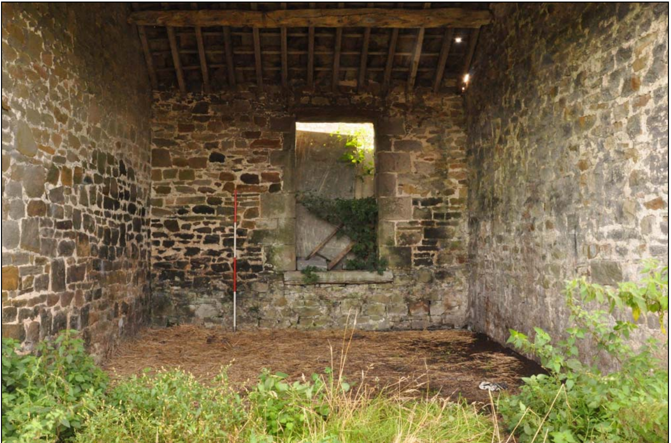
Photo 29: South-west bay in outbuilding, from the north-west
