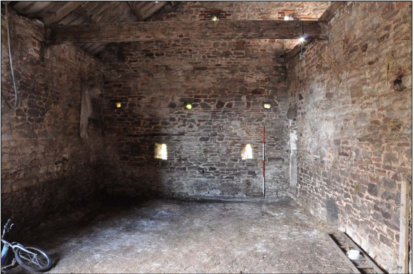
Photo 7: Interior of original barn, from the north-west
