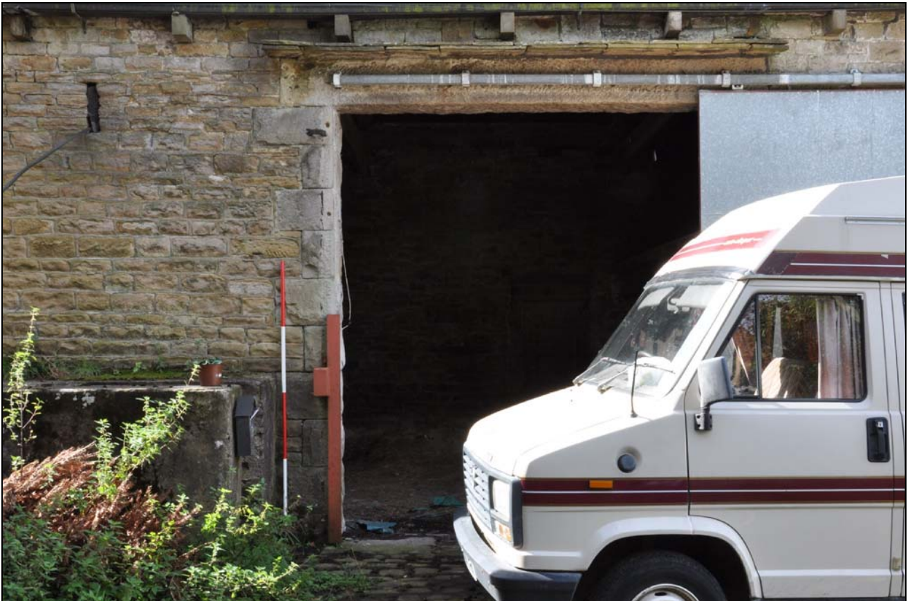
Photo 4: Cart doorway in north-east side of barn
