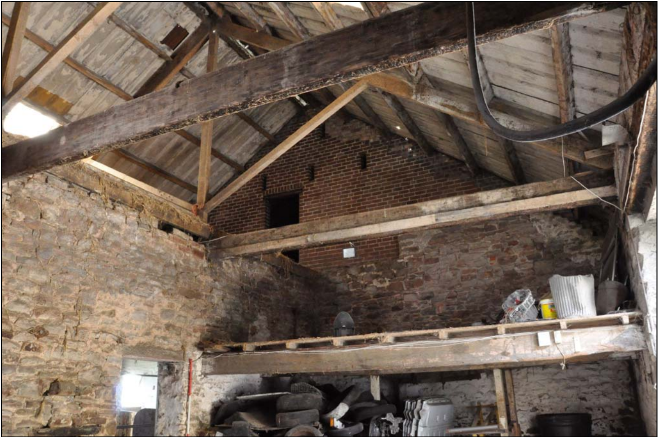
Photo 11: View up towards roof, from east corner of barn
