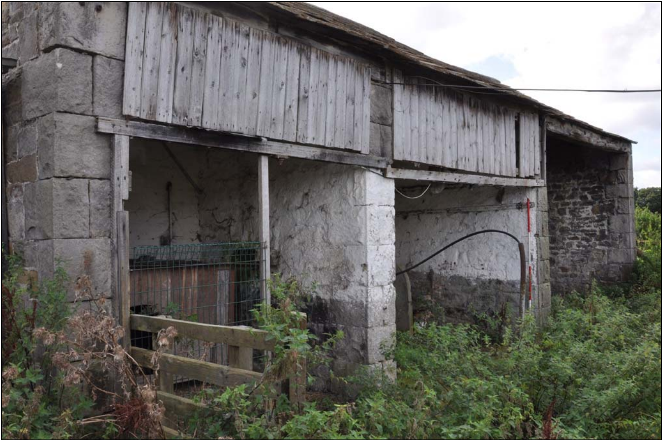
Photo 28: The outbuilding, from the north
