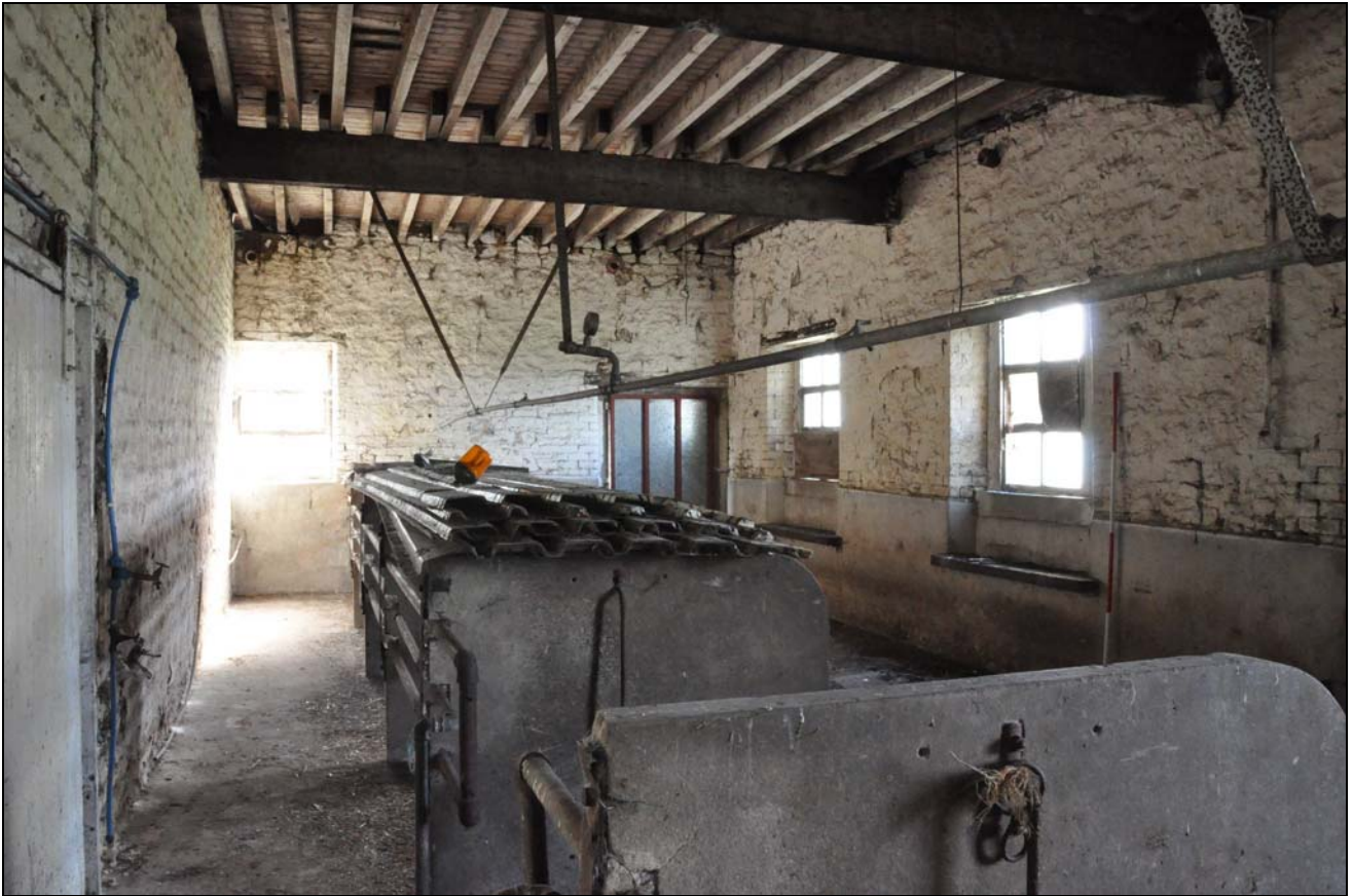
Photo 20: Large shippon in south-west side of barn, from the north-west
