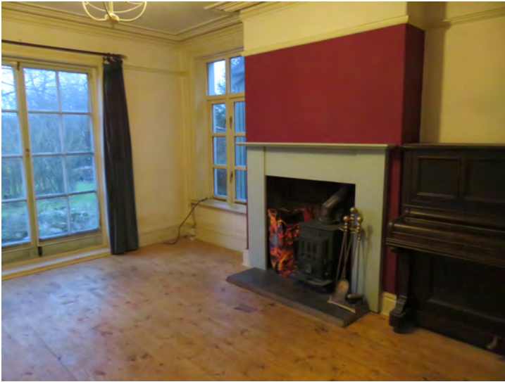
Interior view of existing Dining Room.
