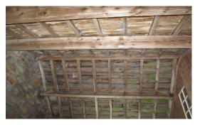
The adjoining barn roofs are unlined and supported by modern bandsawn trusses.
