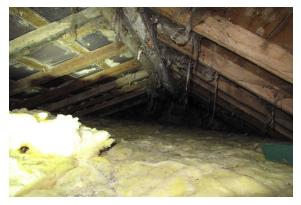
The loft of the farm house is insulated. The slates are unlined and exposed and flight space withing the loft is limited. Both loft spaces are heavily cobwebbed.
