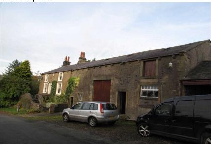
The property is two storey traditional stone built semi detached house with double pitched slate roof, Stonework and rendering is in good condition, and pointing is good with no obvious crevices, gaps or cracks present.
