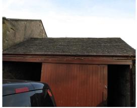
The roofs of the house and barn are in generally good condition with no lifted slates or gaps between slates present, ridge tiles have some pointing missing.
