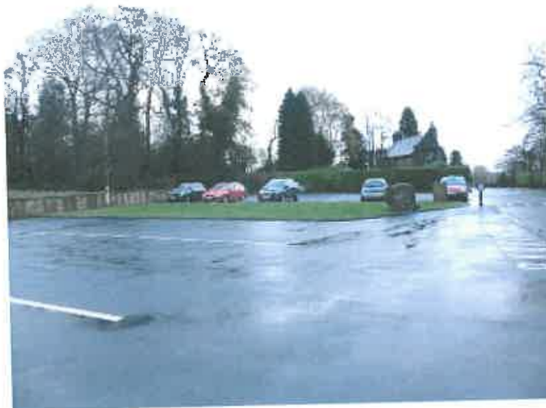
Fig.15: existing car and coach park, from the west
