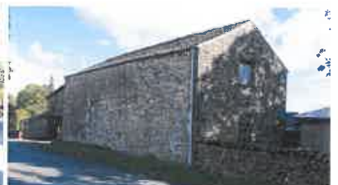
Figure 9: Front (north) elevation Barn 'B'
