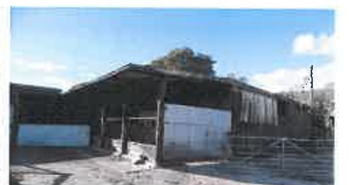
Figure 15: timber-framed sheds 'E'
