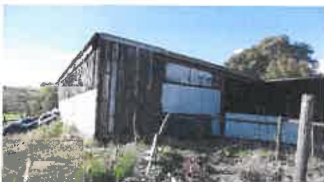
Figure 14: steel-framed shed 'E'
