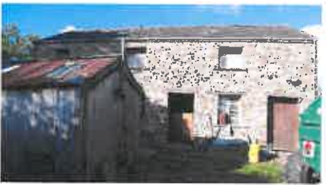
Figure 10: Rear (south) elevation barn 'B'
