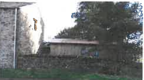
Figure 13: Cubicle shed 'C'
