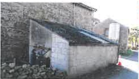
Figure 8: Lean-to shed /dairy on Barn 'A'
