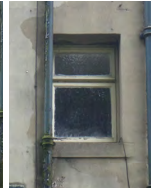
ix) Window WF.5 - First floor, No. 17 - rear elevation.
