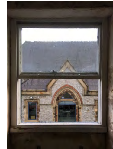
iv) Internal view of window WS.2 - Second floor, No. 17.
