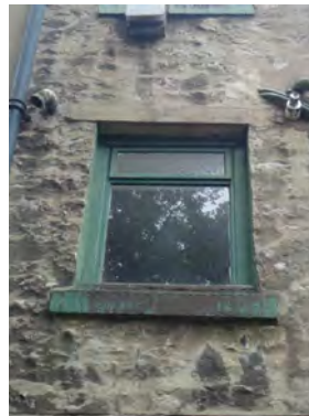
x) Window WF.6 - First floor, No. 15 - rear elevation.
