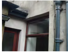
vi) Window WG.5 - Ground floor, No. 17 - rear elevation.
