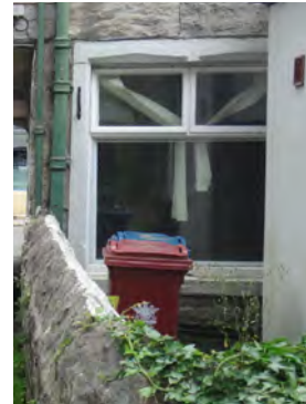
vii) Window WG.6 - Ground floor, No. 15 - rear elevation.
