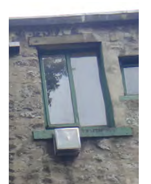
xiii) Window WS.5 - Second floor, No. 15 - rear elevation.
