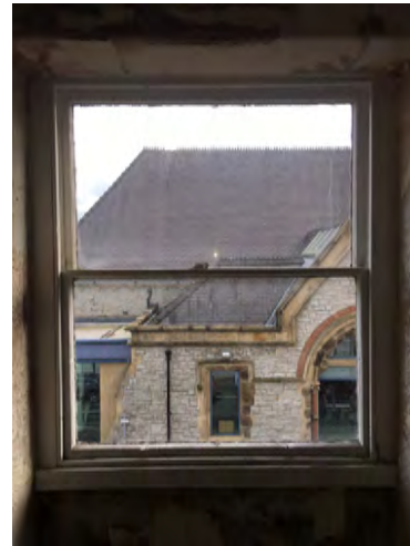
iii) Internal view of window WS.3 - Second floor, No. 17.
