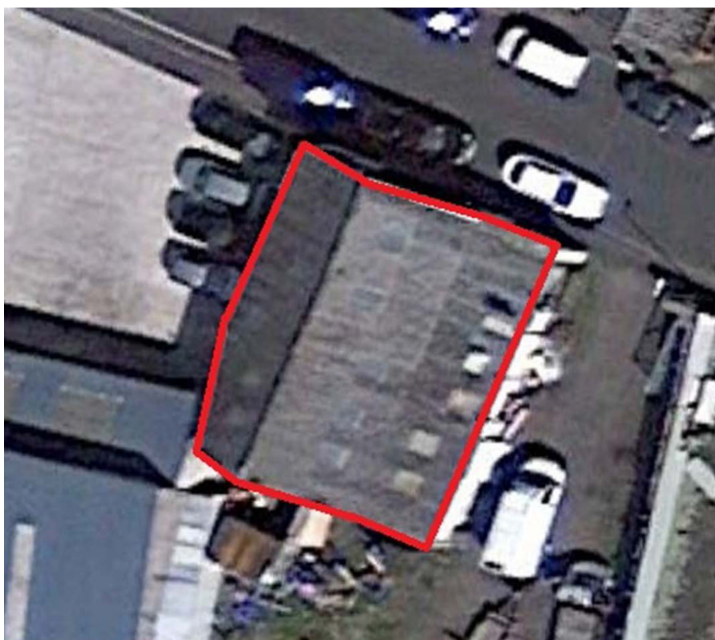
Aerial Image - Roof area to be replaced highlighted.
