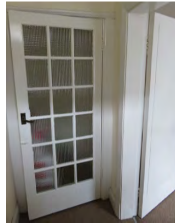
xvi) Number 17 - item 17 - front entrance lobby.
