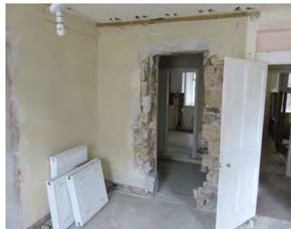
xiii) Number 15 - item 14 - opening between first floor existing bathroom and Number 17.
