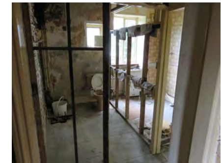
xv) Number 15 - item 16 - late-C20th stud partitions to second floor rear right room.
