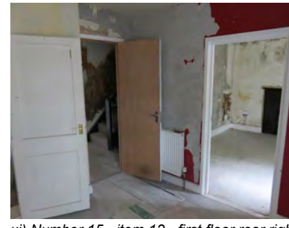
xi) Number 15 - item 12 - first floor rear right room.
