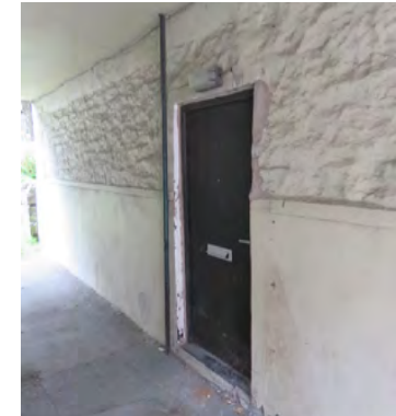
xix) Number 17 - item 20 - entrance to upper flats off passage.
