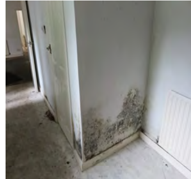
iii) Number 15 - item 6 - modern partitions to rear kitchen.
