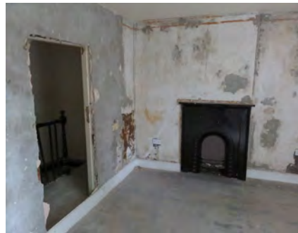
x) Number 15 - item 11 - opening from first floor landing to rear left room.
