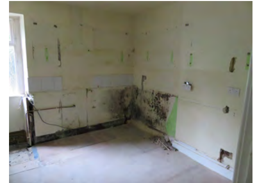
xxiii) Number 17 - item 26 - existing first floor kitchen.
