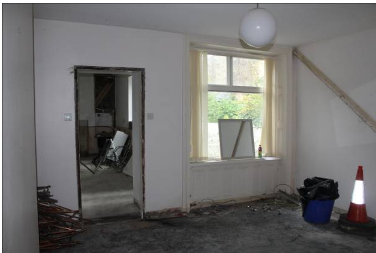
15. Rear ground floor room of 15, with late 19 th century window and panelling
