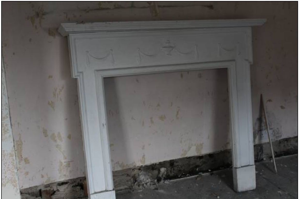
22. Adam-style fire surround in first floor front room of 17
