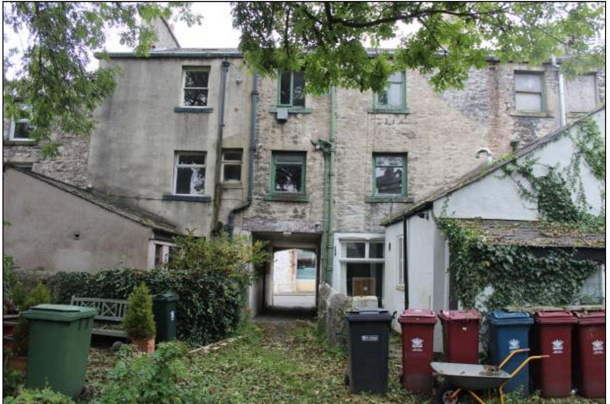
7. Rear of the buildings, viewed from the enclosed yard
