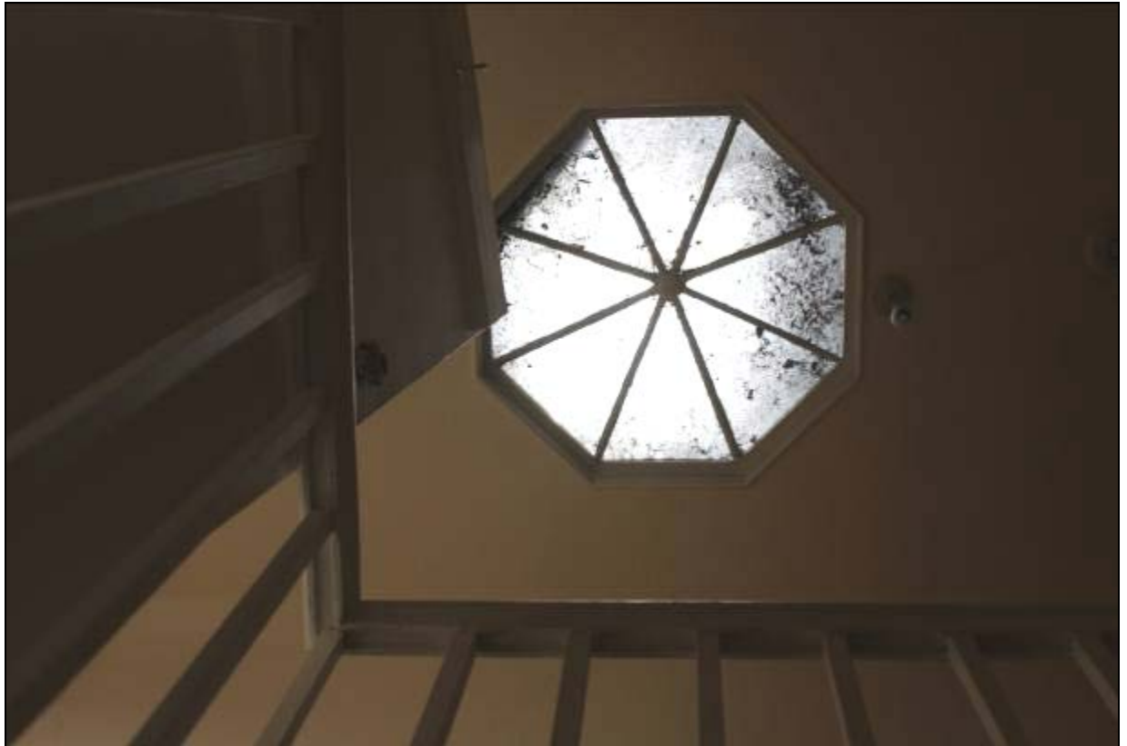
24. Overlight to stairwell of 17
