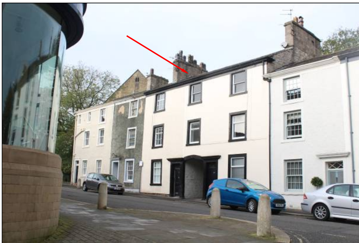
1. The application buildings (indicated), looking northwest into York Street
