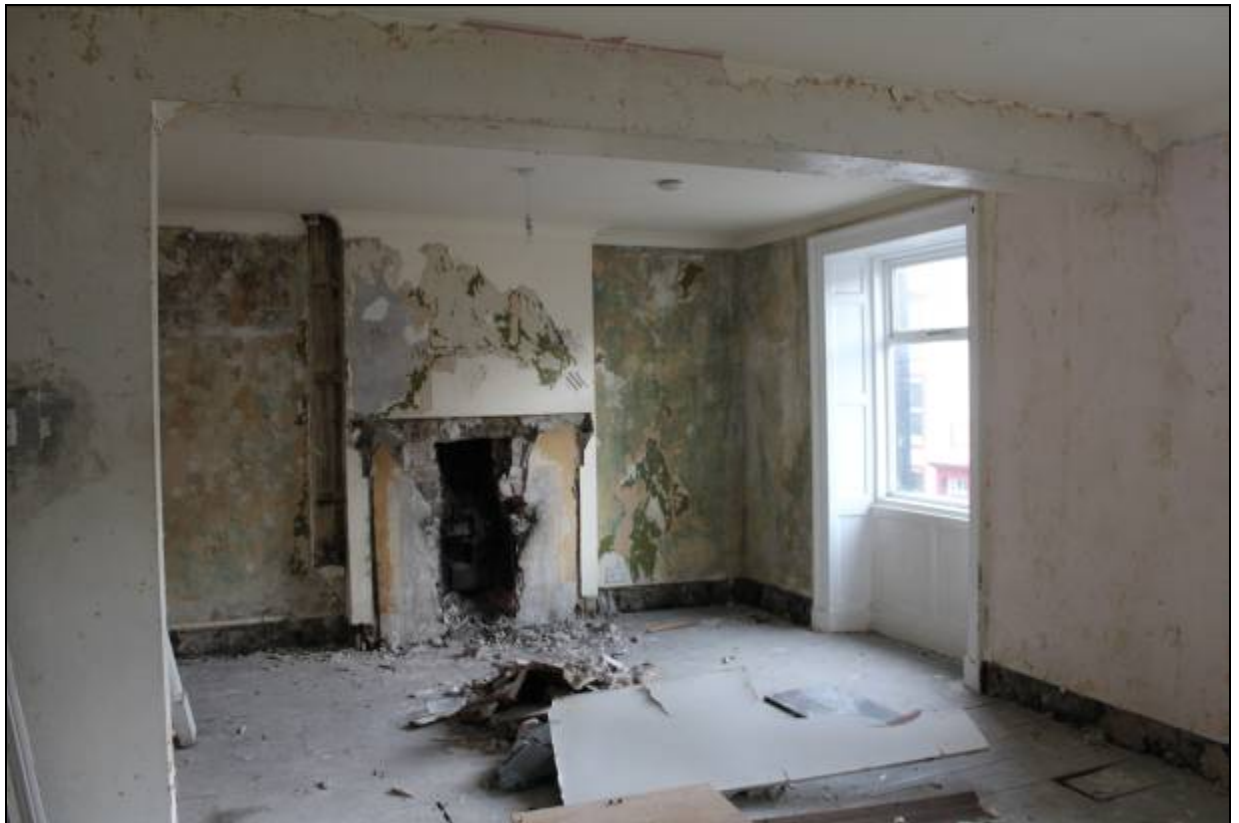
20. First floor front room of 17, showing removed crosswall
