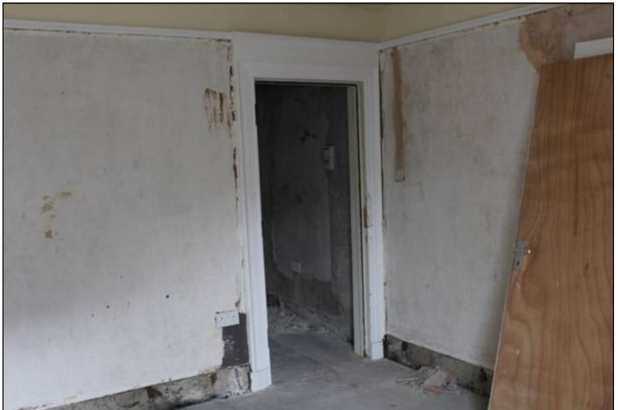
19. Door architrave in first floor front room of 15
