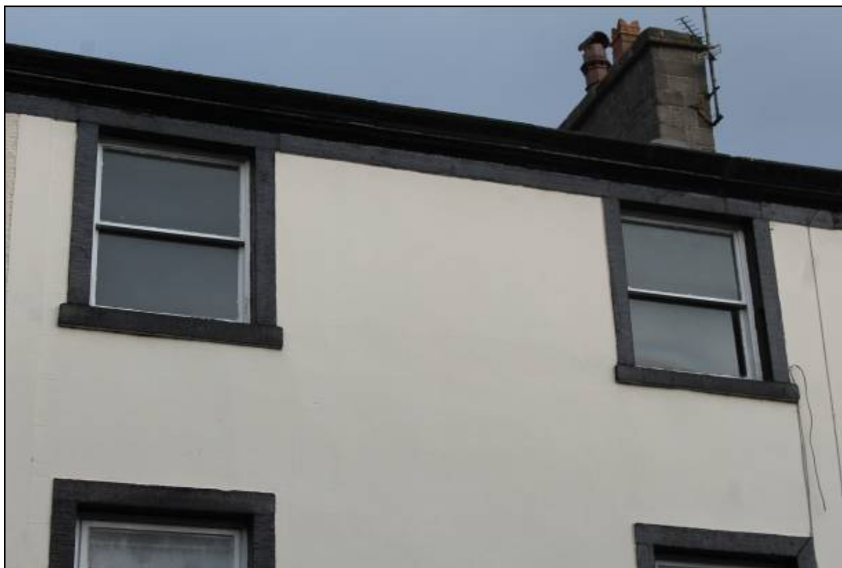
5. Sash windows on second floor of 17, large panes indicating they are not original
