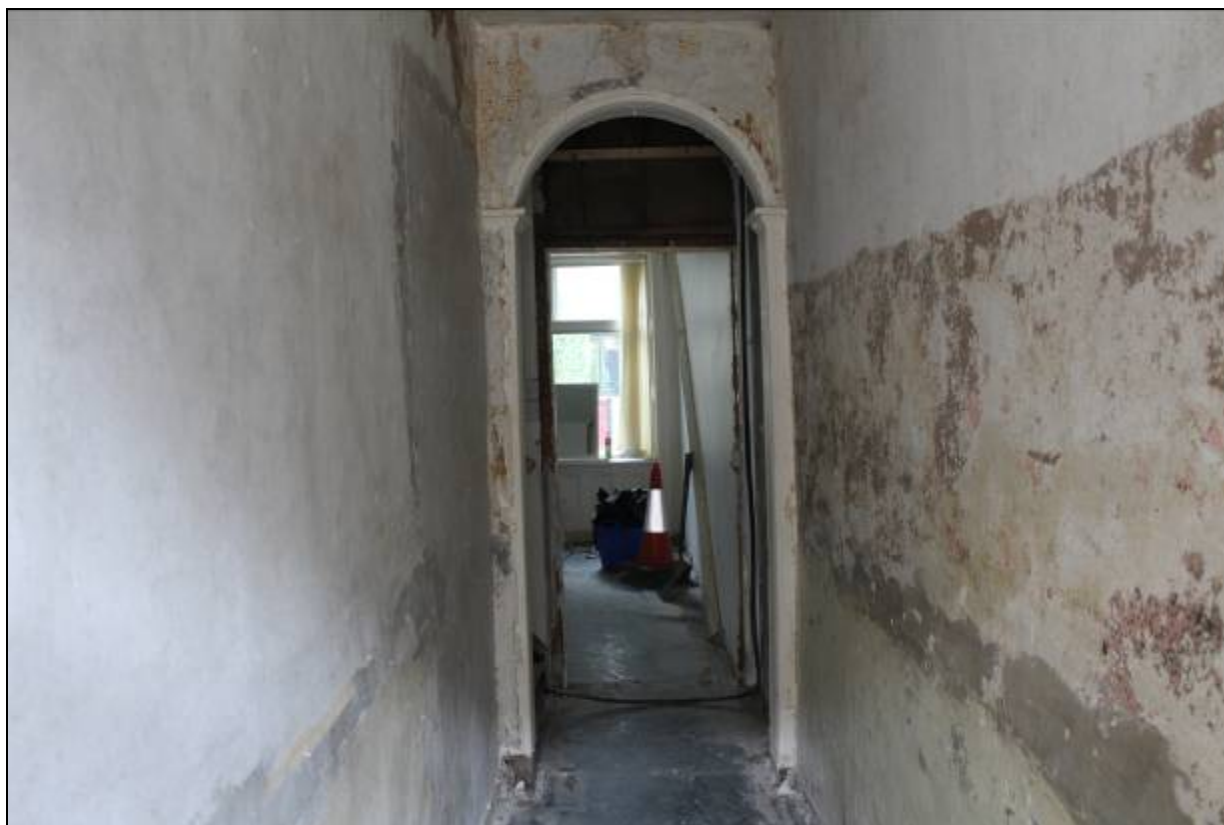
14. Entrance hallway to 15: blocked door to front room on left
