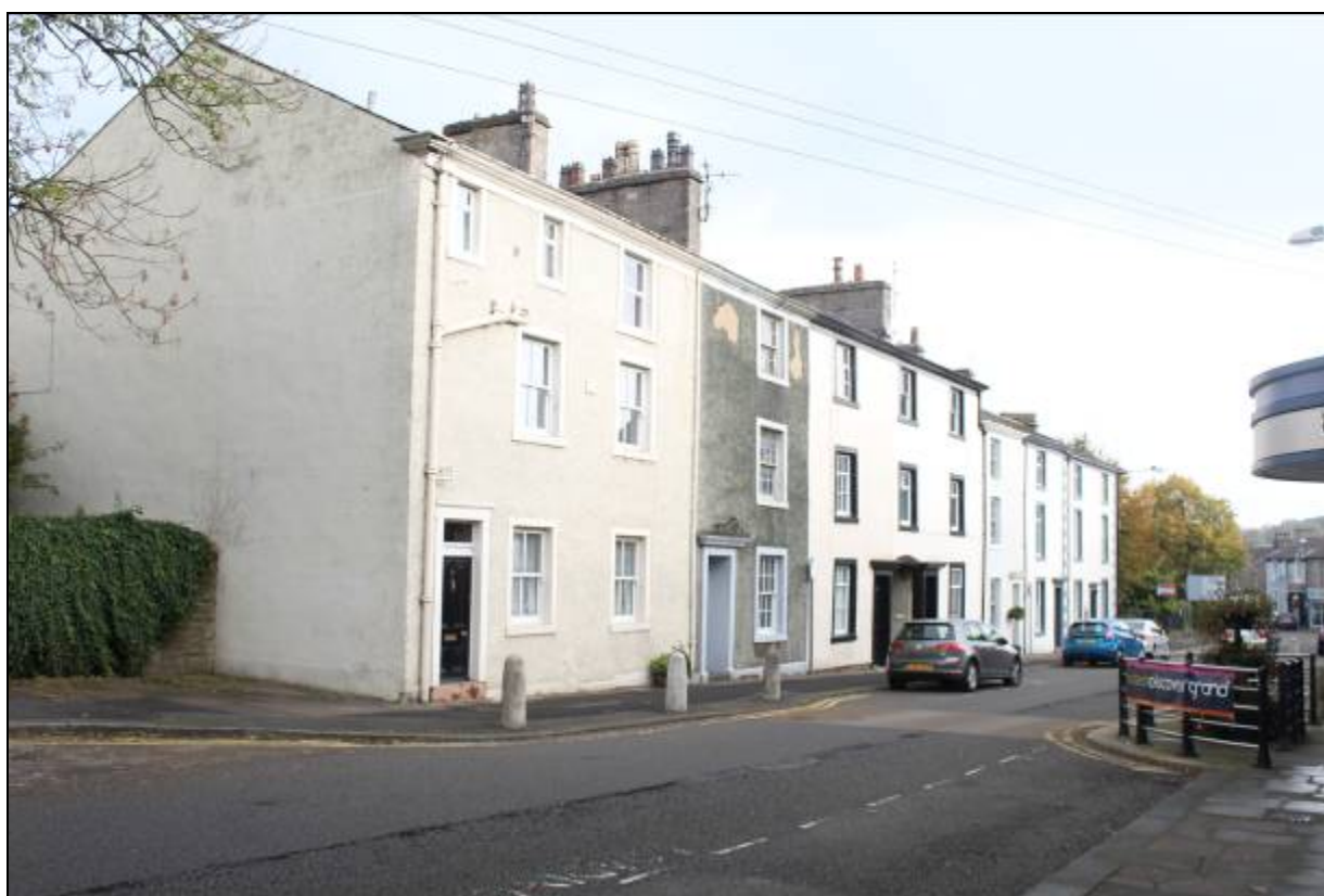
2. The terrace of which the buildings form part, looking northeast along York Street
