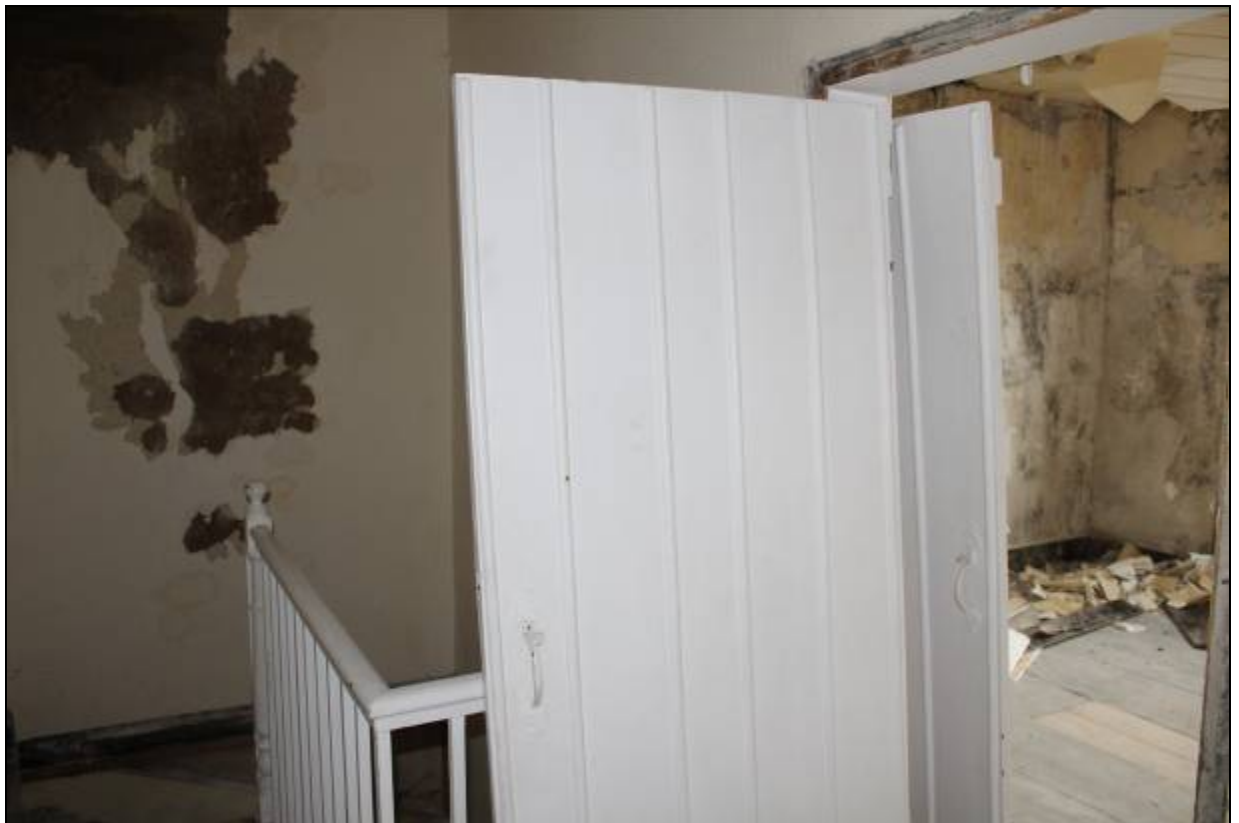
25. Batten-plank doors to second floor of 17, probably circa 1900
