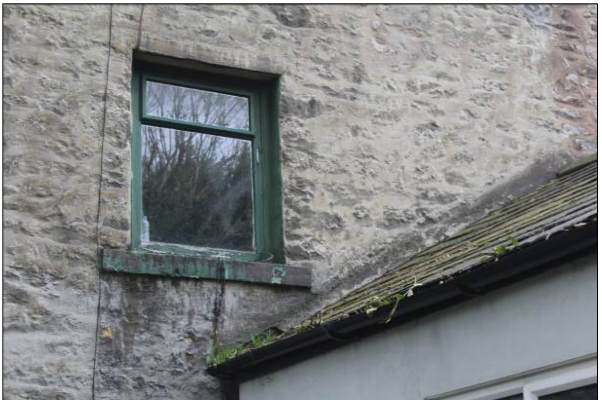
8. Example of mid-20 th century casement at rear of 15
