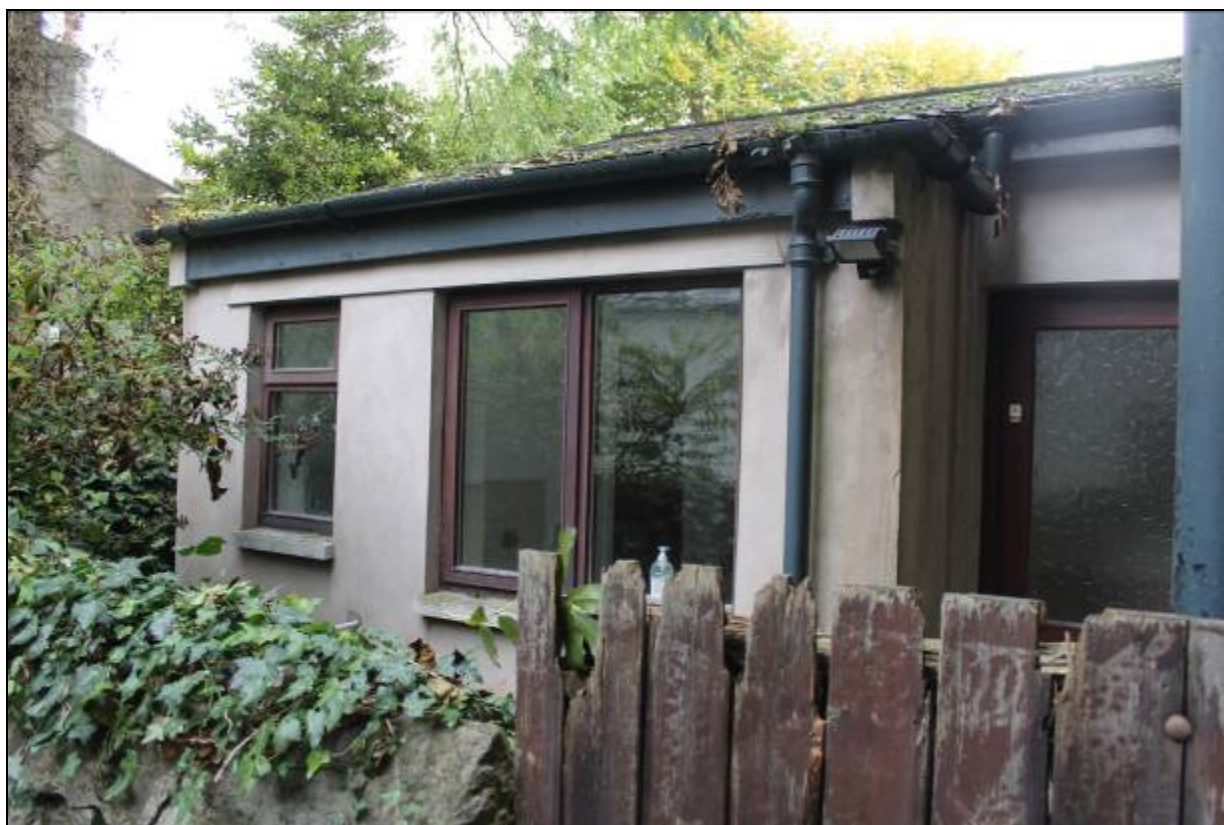
10. Outrigger to rear of 17 was rebuilt in 1996
