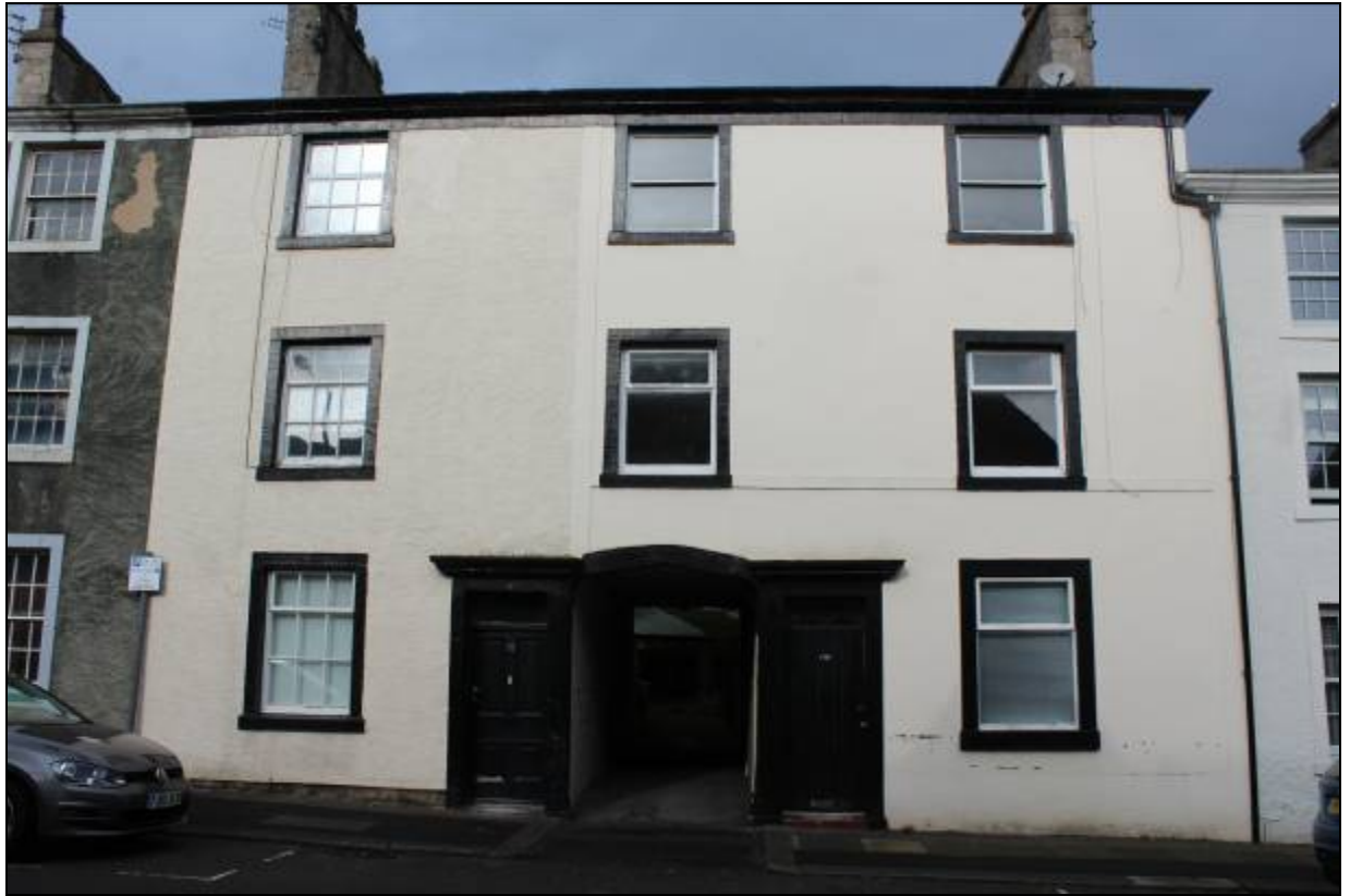
3. Front elevation of the buildings to York Street
