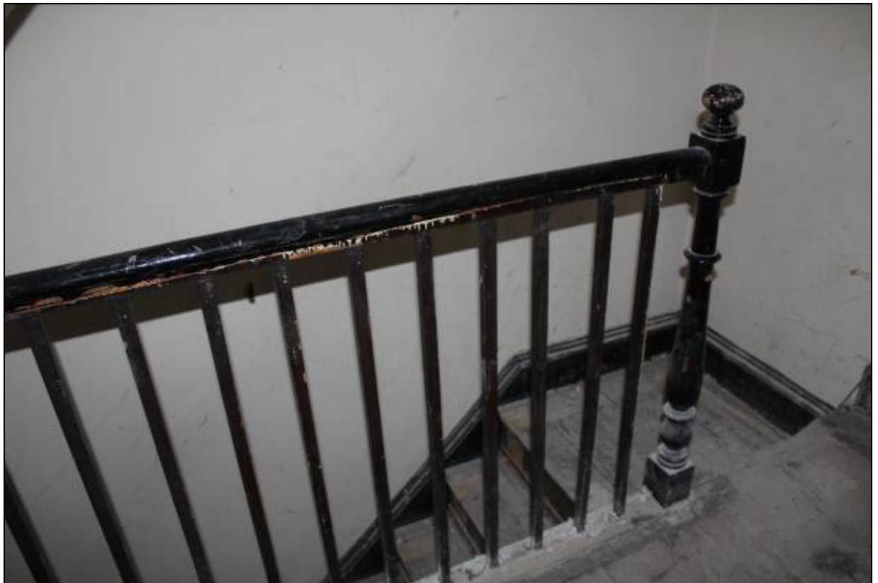
16. Original stair at first floor landing of 15
