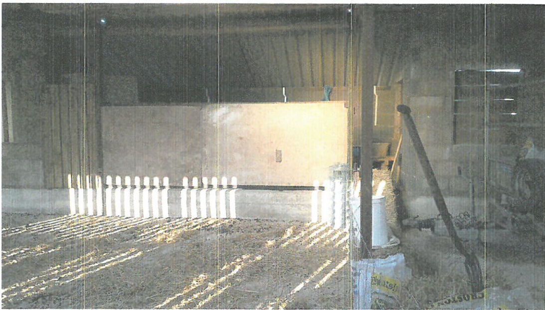
Interior looking north towards outrigger
