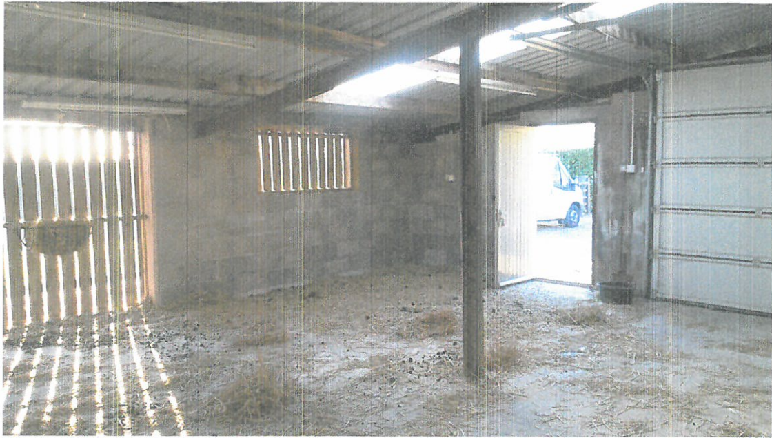
Interior looking south-west
