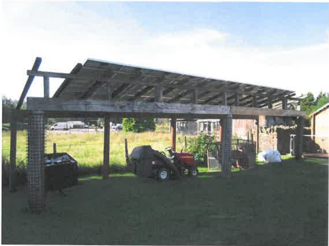
3 Pergola adapted to support solar panels.
