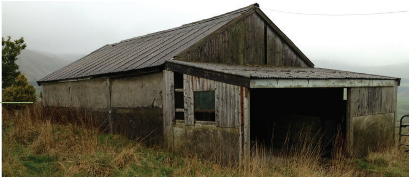
EXISTING SHED TO THE NORTH TO BE DEMOLISHED
