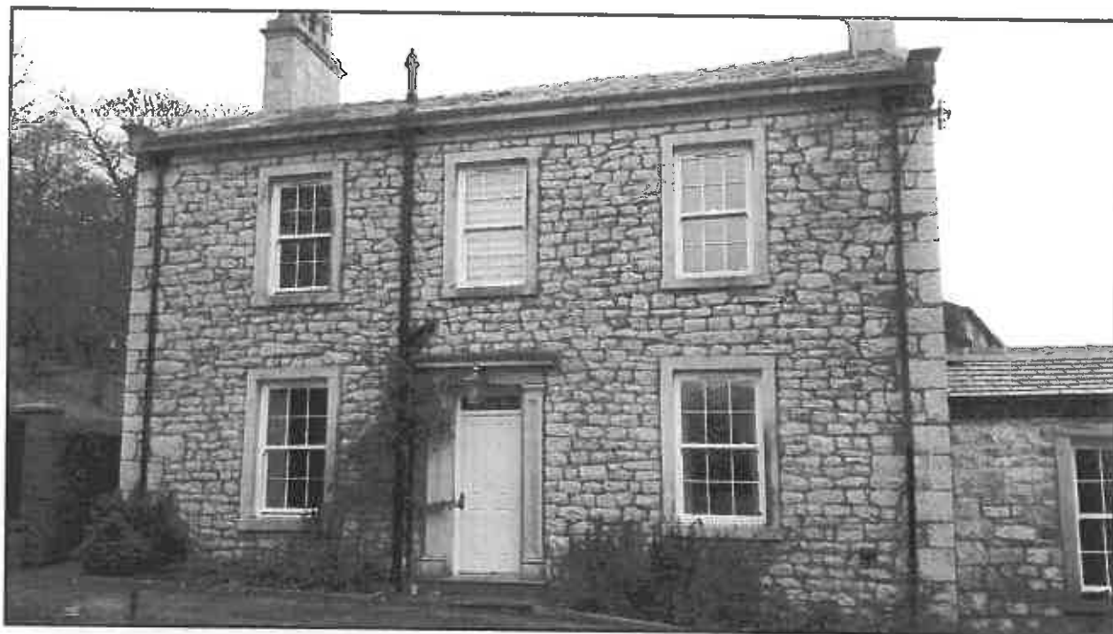
Figure 2) Holmes Cottage, west facing elevation
