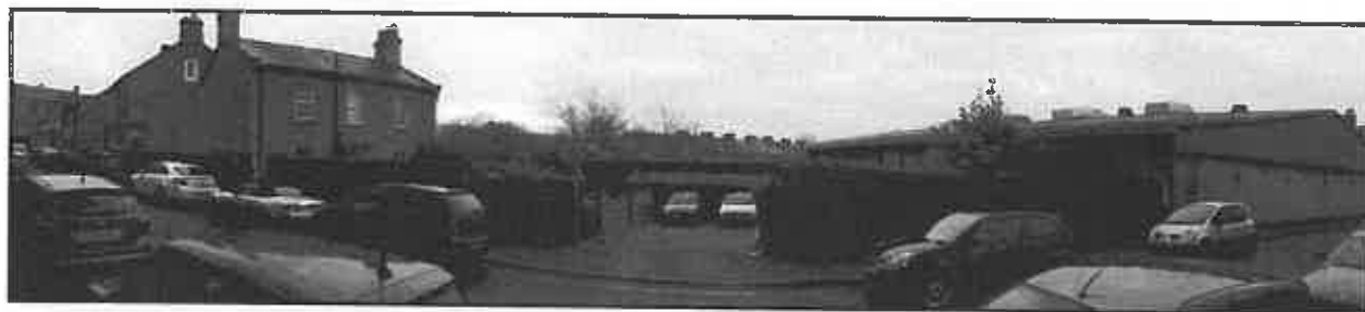
Figure 3) Panoramic view from Woone Lane showing Cottage (left) and neighbouring Mill buildings
