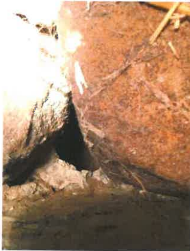
Plate 9: The stone walls had areas of missing pointing allowing access within.
