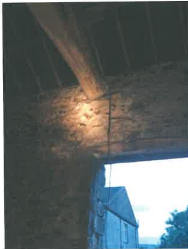
Plate 11: Numerous gaps were present in the walls around the wooden roof frameworks.
