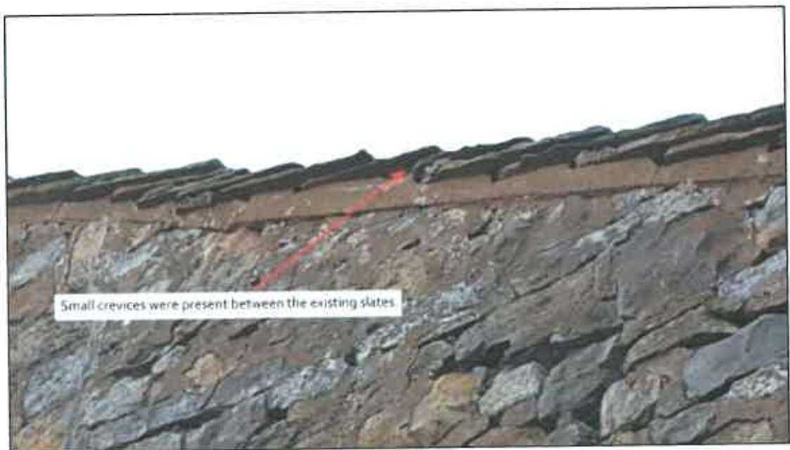
Plate 4: All along the roof verges there were numerous possibilities for bats to gain access to possible bat roosting locations.
