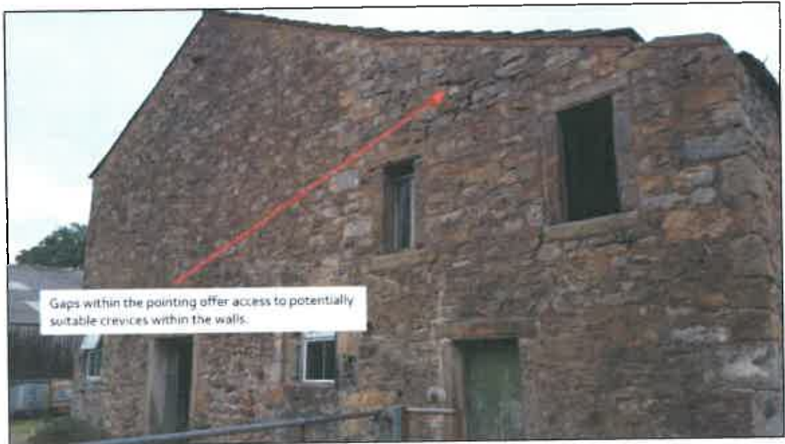
Plate 3: The southern aspect of the western barn. Abundant gaps in the walls could be found on this aspect and others. In addition, many of the entrance (i.e. windows and door) were completely open to the elements.
